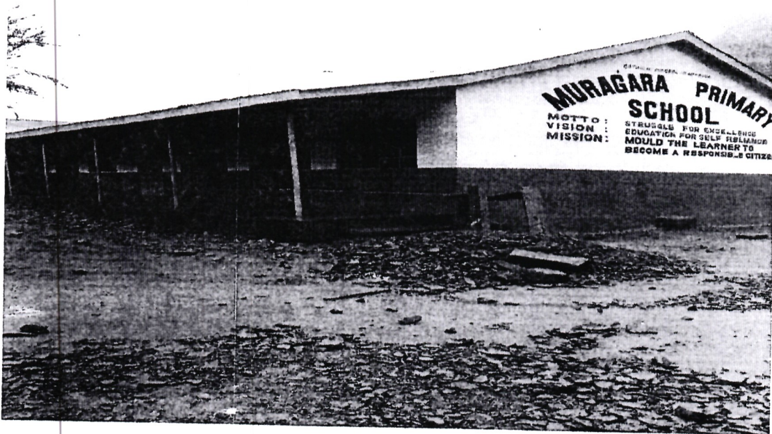
Muragara primary school renovation of classrooms
