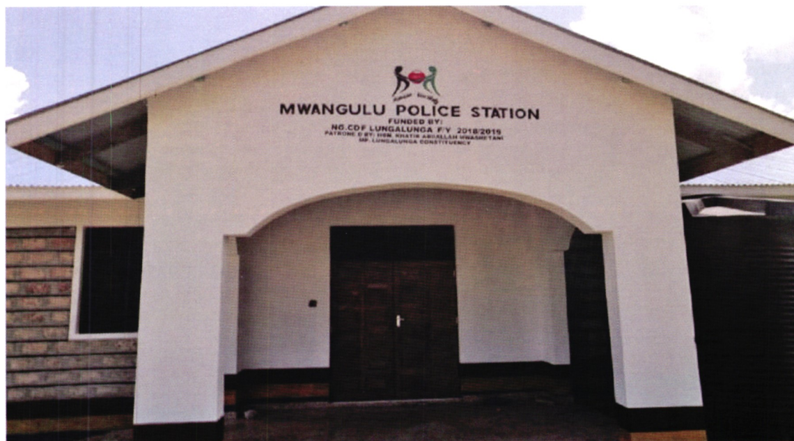
Photo 1: Offices under construction at Mwangulu Police Station, which are funded by NG-CDF Lungalunga
