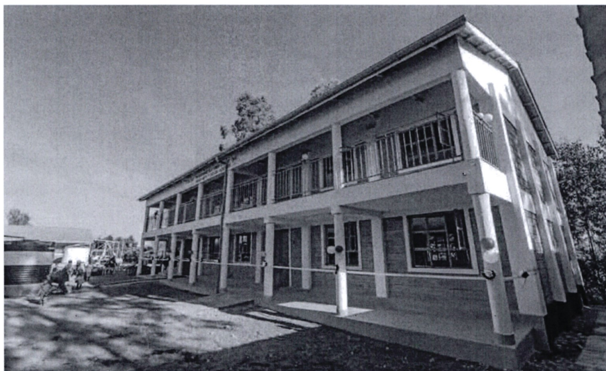
Ilmerijo Primary School, Construction of a 4 No classroom block
