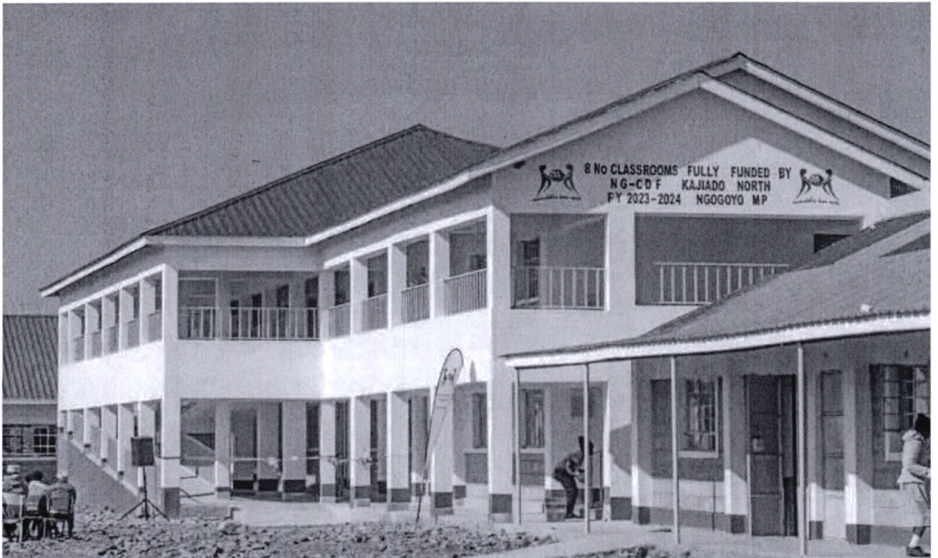
Embulbul Primary School construction of 8No. classrooms fully implemented in the 24/25FY
