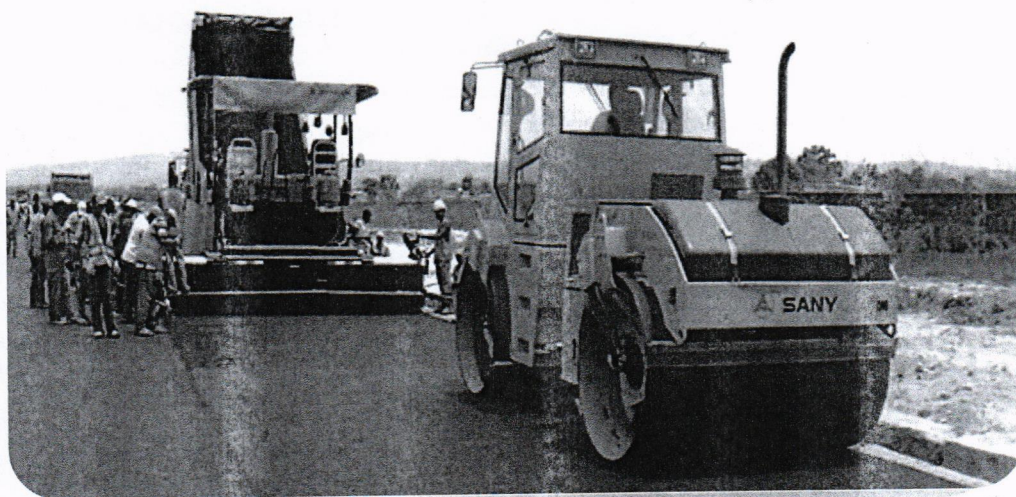
Figure 6: Road Maintenance Project in Progress
