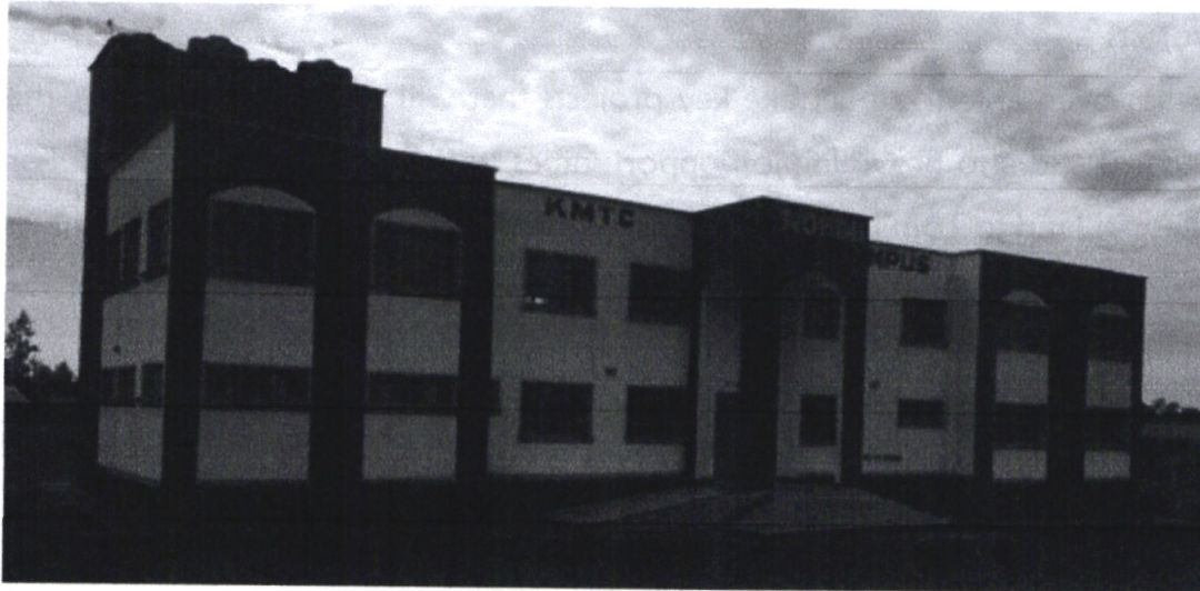
Construction to completion of Ndhiwa KMTc
