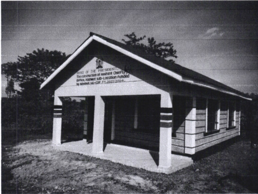
Fig 1: Construction to completion of kaduet Assisatnt Chiefs Office
