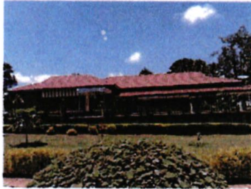
Refurbishment and operationalization of a staff's canteen
