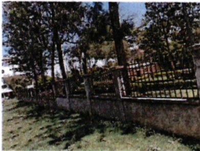
Construction of a perimeter wall
