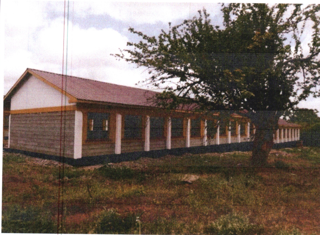
Kenya Medical Training College Tseikuru- Construction of 10 classrooms to completion
