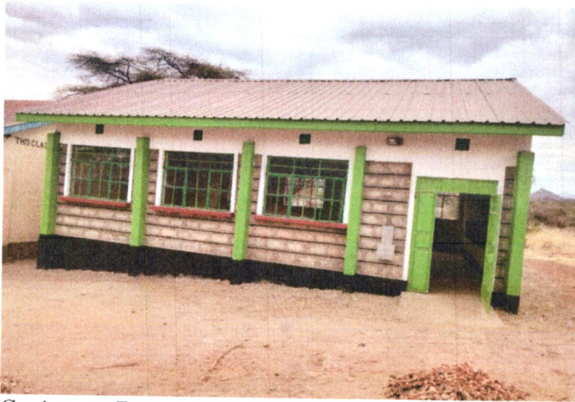
Gacigongo Primary School- Construction of 1 classroom to completion
