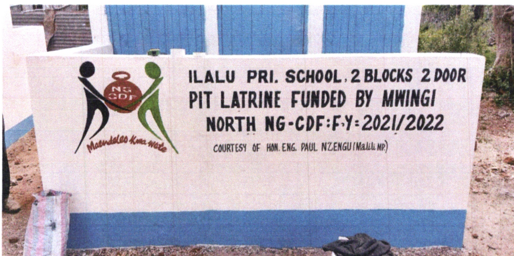
Ilalu primary school- Construction of 2No. blocks of 2 door pit latrines
