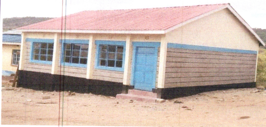
Malili Primary School- Construction of 1 classroom to completion
