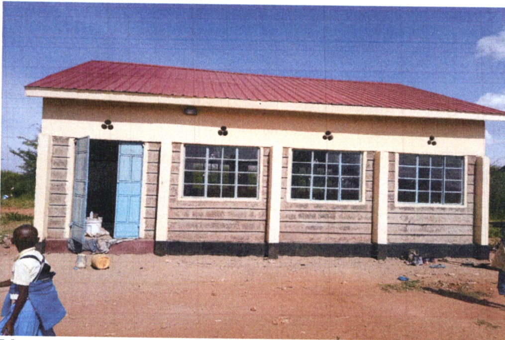
Ithunzi Primary School- Construction of 1 classroom to completion
