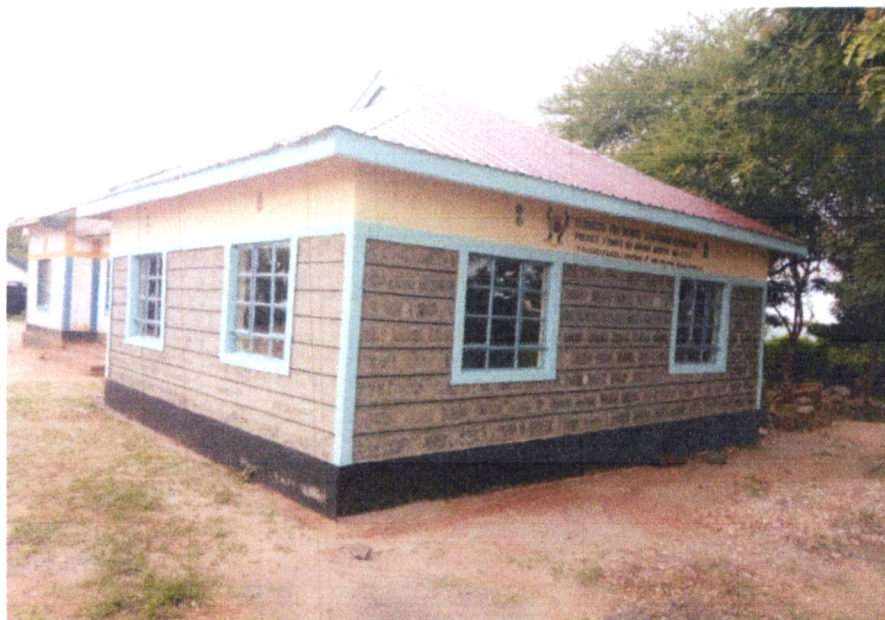
Itivanzou Primary School- Construction of an extended 1 roomed administration block to completion
