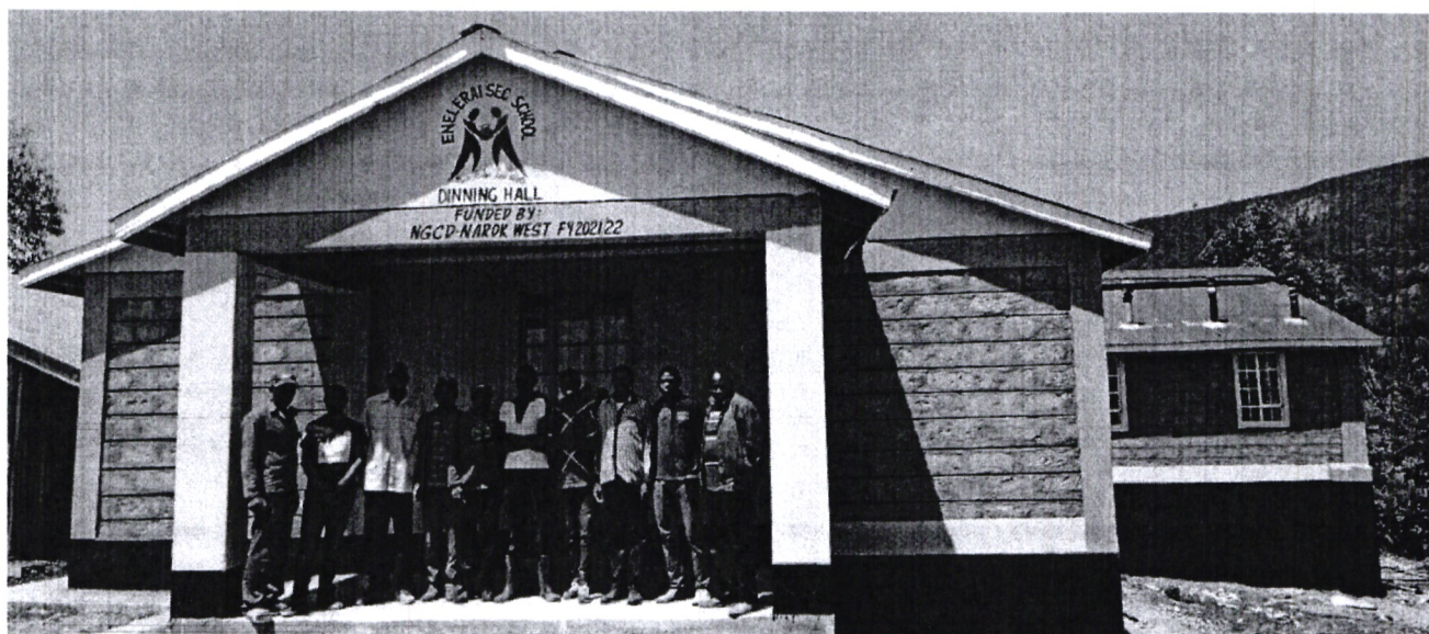
Enlerai Secondary School: Construction of a 45-student capacity Dining Hall to completion.
