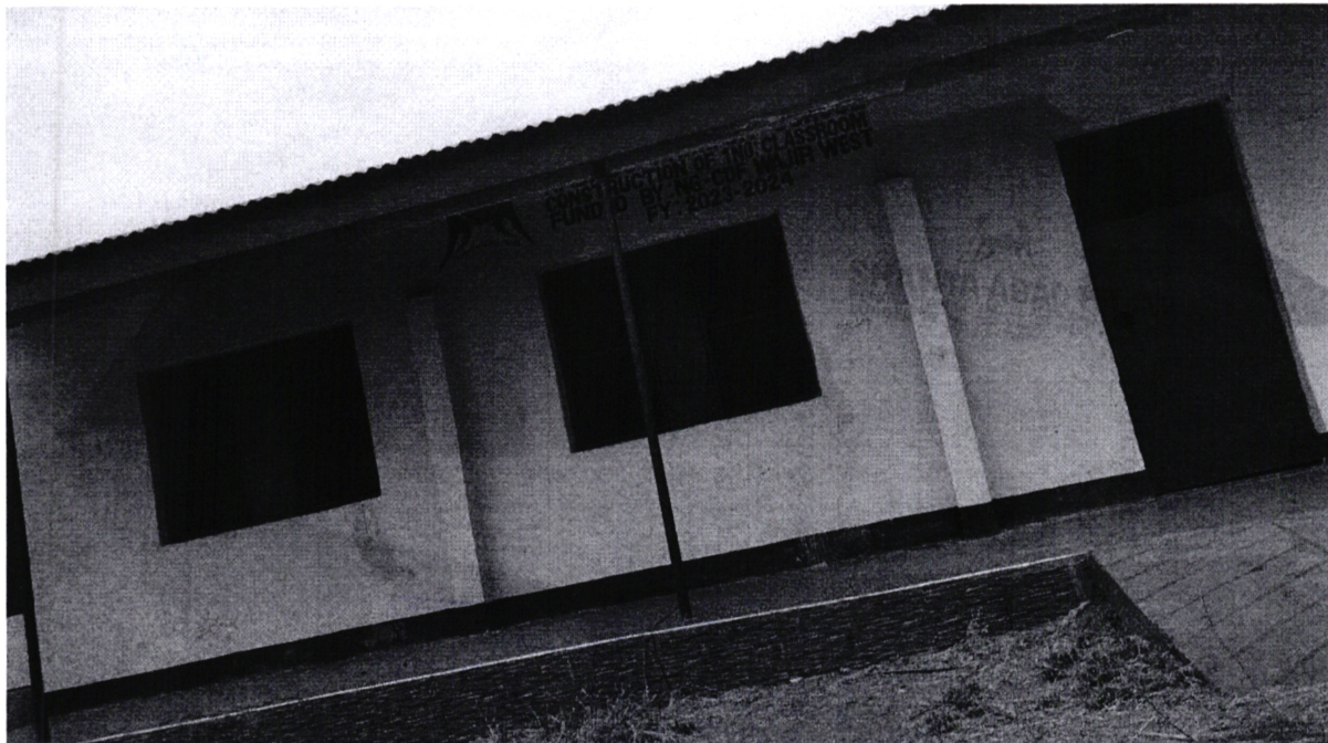
Hadado Secondary School is situated in Hadado location, Hadado/ Athlbohoh ward. It is a mixed day and Boarding secondary school. It has a student population of 900 students. Wajir West NGCDF has funded the construction of an additional classroom to accommodate the increasing population of students.
