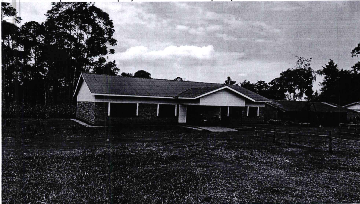
SHAGUNGU PRIMARY SCHOOL ADMINISTRATION BLOCK
