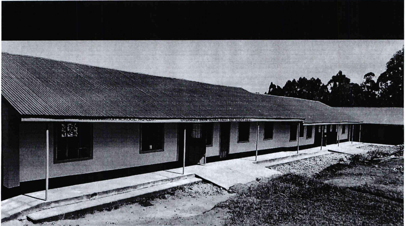
RENOVATION OF 8 CLASSROOMS AT SHIKUSA GK. PRIMARI SCHOOL. HON. IKANA DELIVERS.
