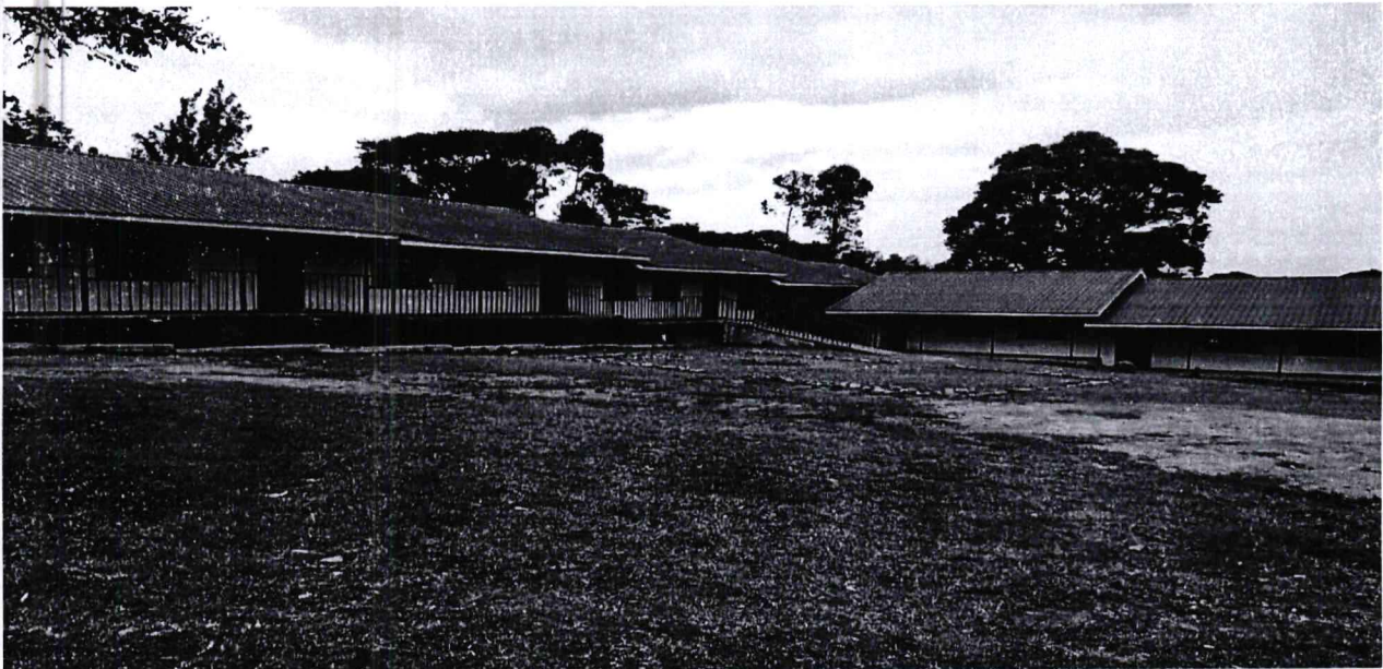
SHILONGO PRIMARY SCHOOL EIGHT NUMBER CLASSROOMS
