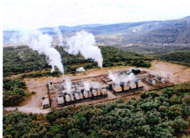
Olkaria Wellhead Generation Plants
