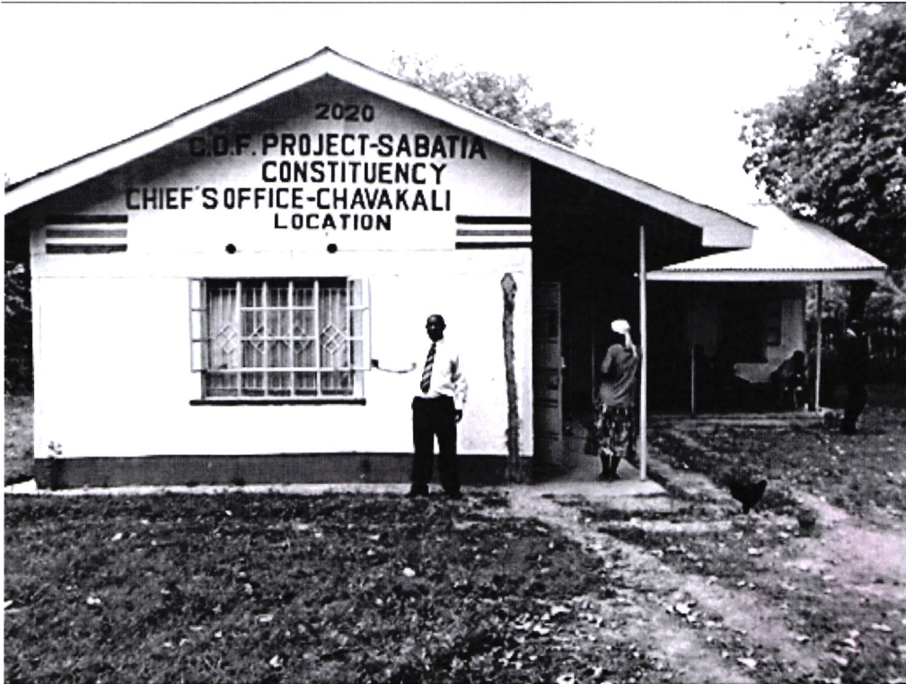
Pic. 2: Construction of Chiefs Office - Chavakali Location funded by Sabatia NG-CDF
