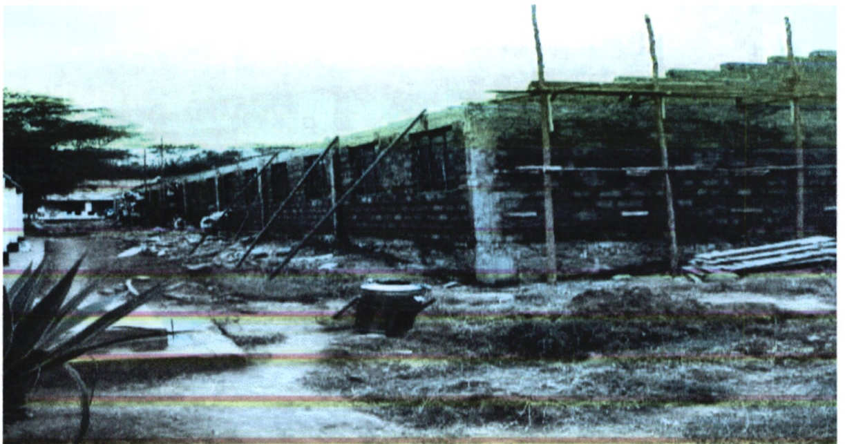
New Hostel Under Construction
