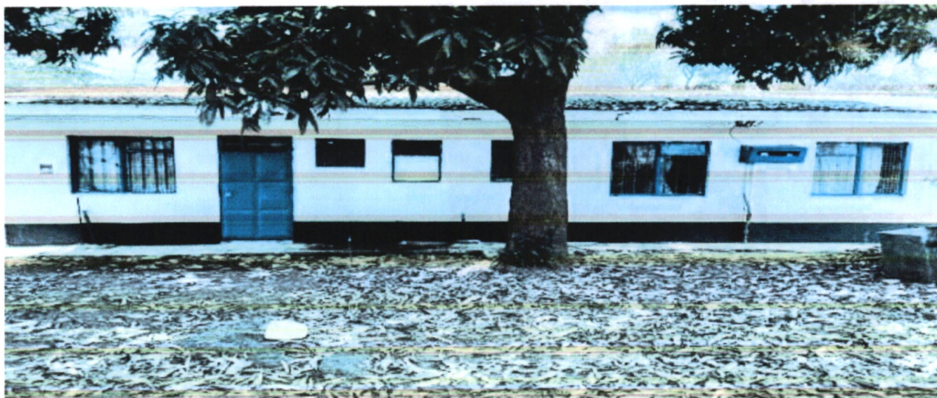
Two (2) staff houses were renovated
