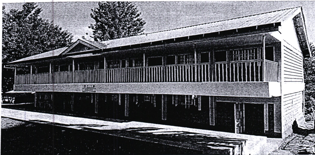
Kiuu Primary School- 2 Classes/Administration Block
