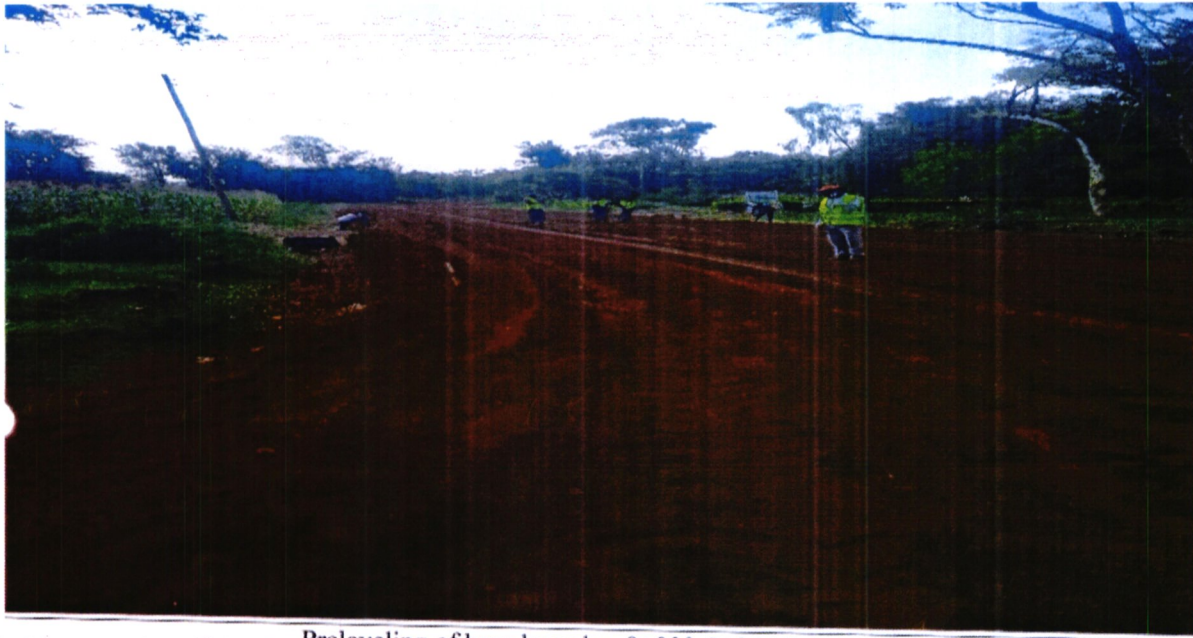
Preleveling of base layer km 0+000-0+264 link 4
