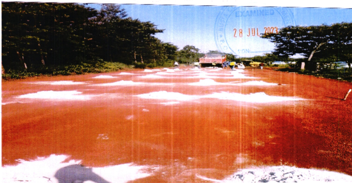
Preleveling of base layer km 0+000-0+264 link 4
