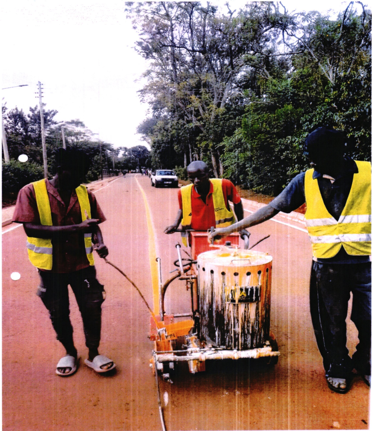
Road Marking in progress
