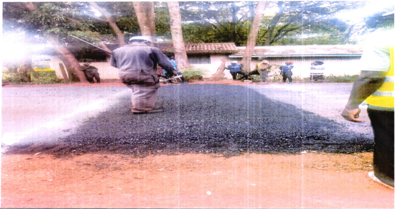
Installation of road bumps at km 0+400 link 3
