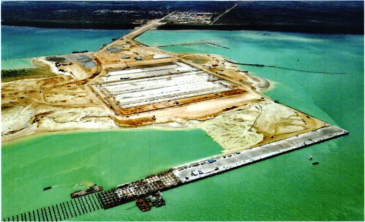
Construction of the first three berths at the New Lamu Port
