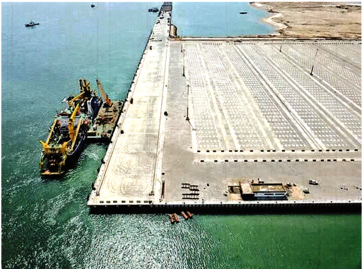
First Berth complete
