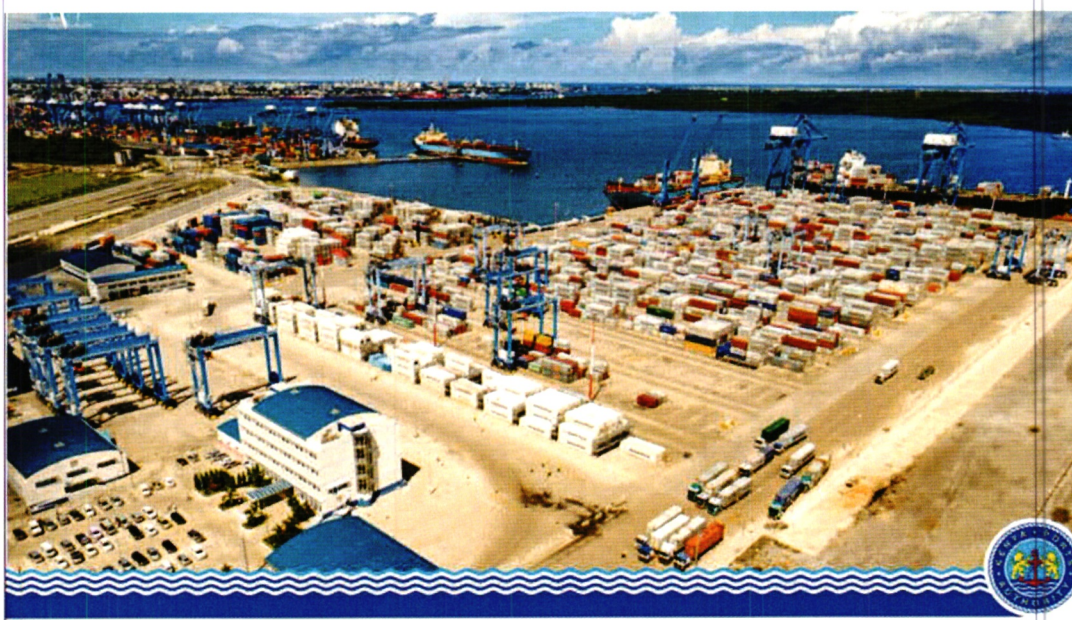
A view of some of the new berths at the Kilindini port in Mombasa
