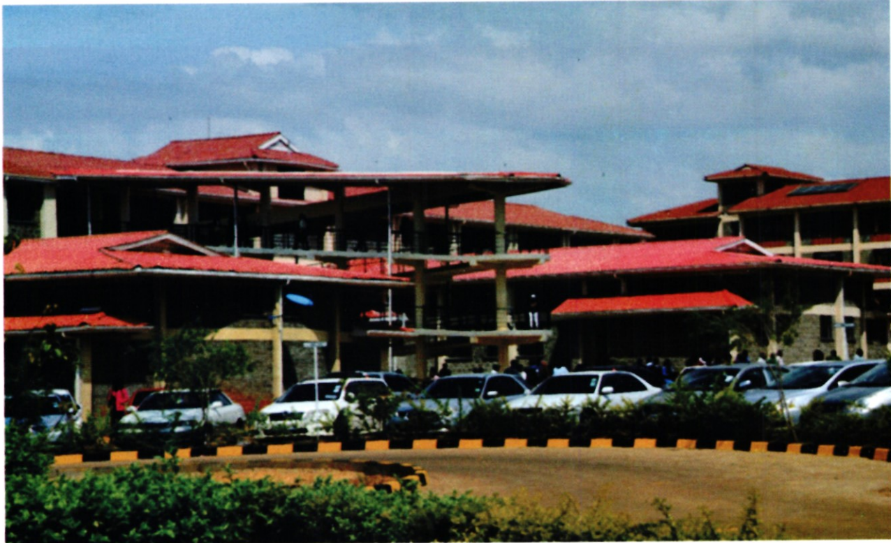
The newly constructed Phase II of the Academic Block complete with a ramp for ease of access by persons with physical challenges
