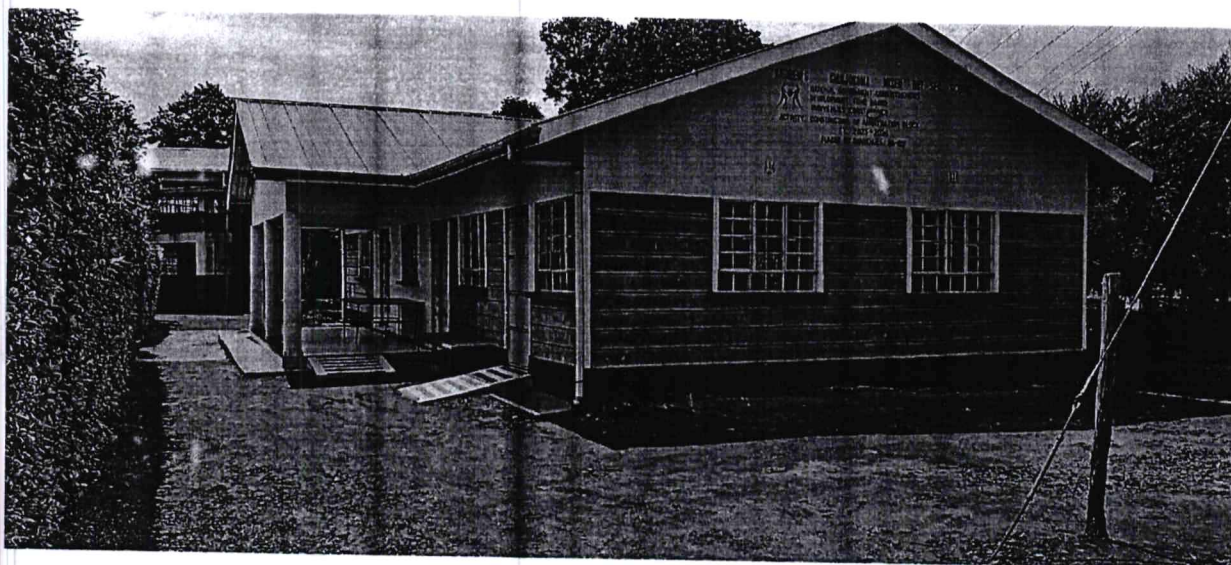
St Andrew Kianjokoma Mixed Secondary School: Construction to completion of an Administration Block
