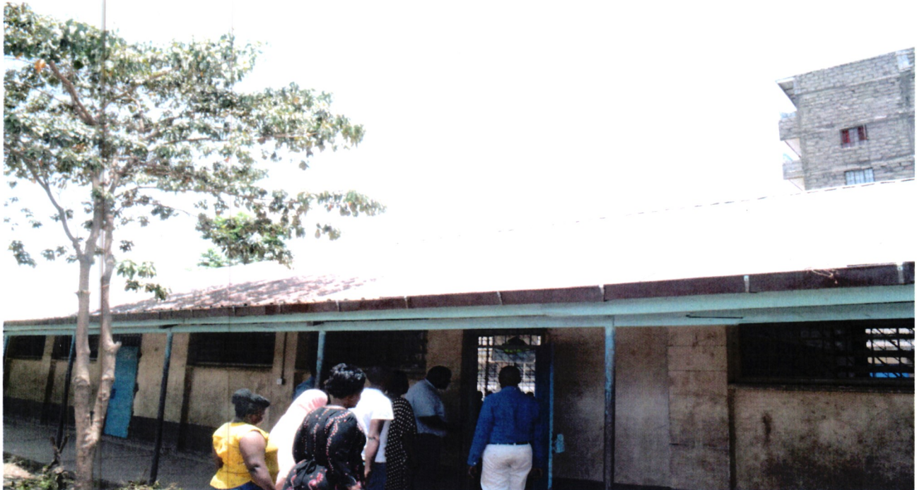
Renovated roof at Martin Luther Primary School
