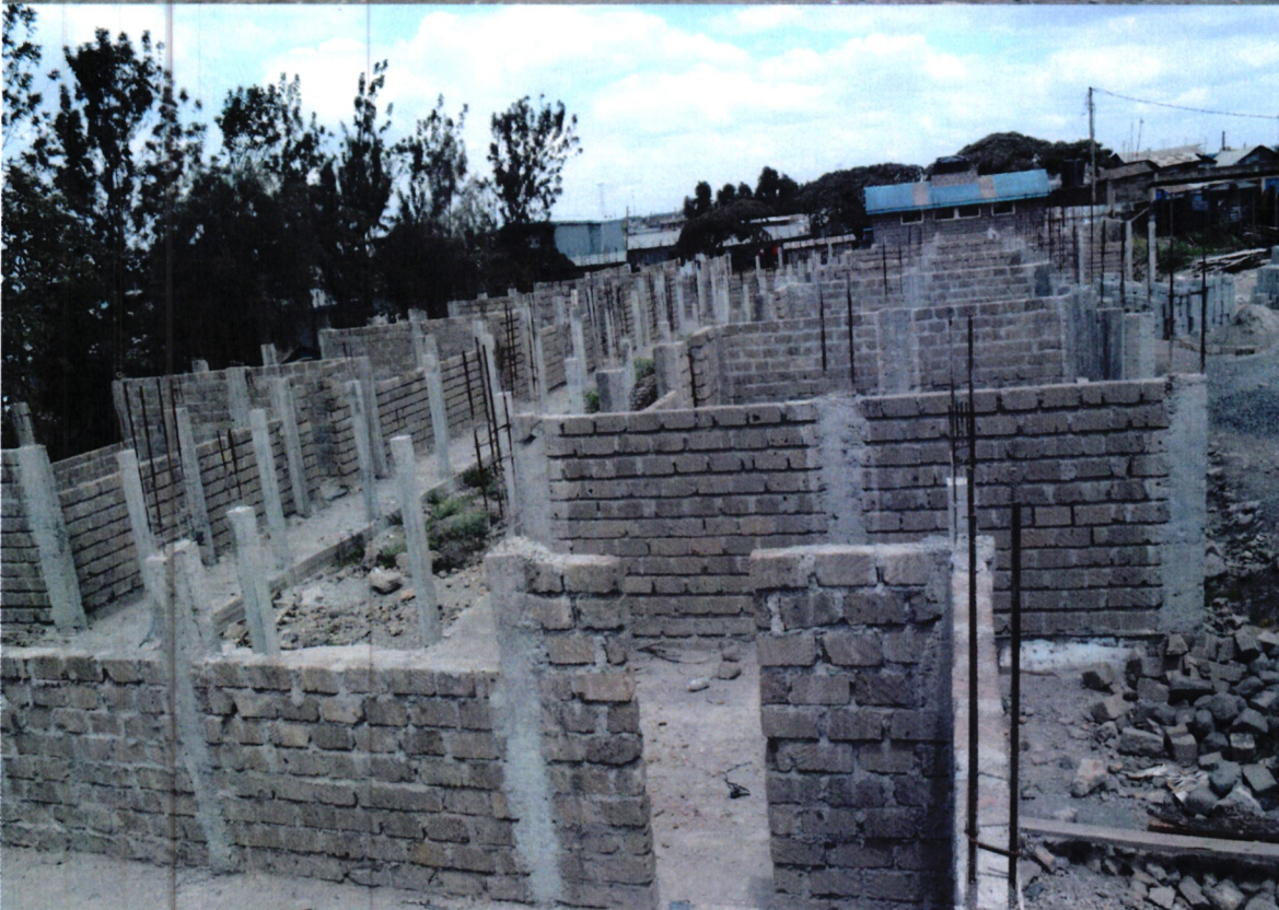
Ongoing Construction of Star of Hope Primary School
