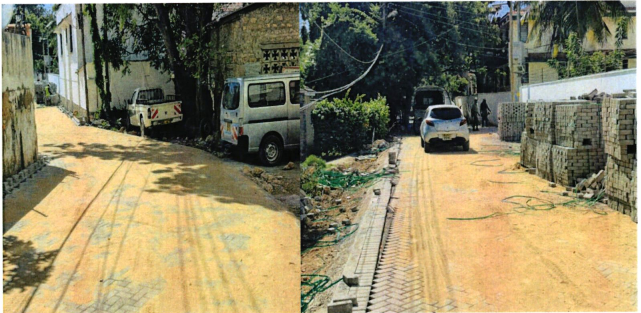
Improvement of Rashid Ali road to cabro Standard, Mvita Sub-County
