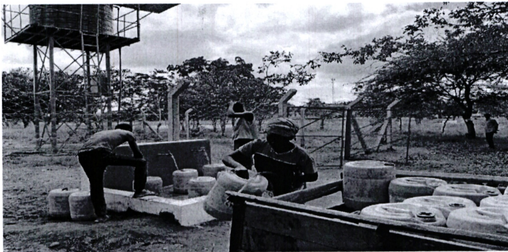
Drilling and equipping Yemulwa borehole in Kathonzweni ward
