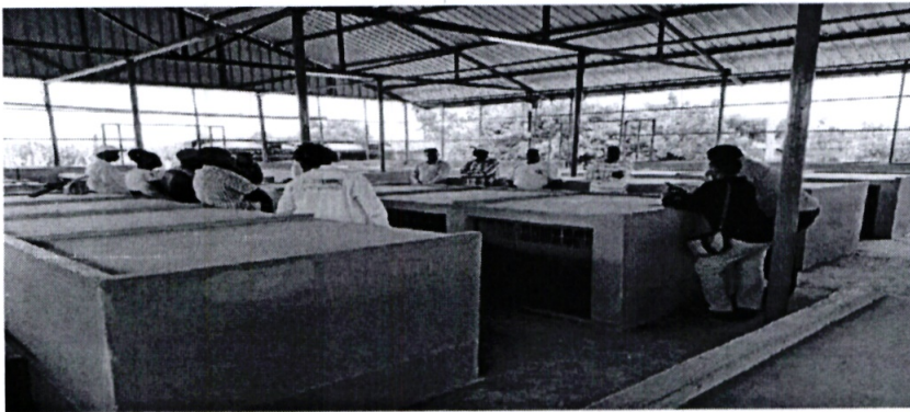
Upgrading Kyanginywa Market shed
