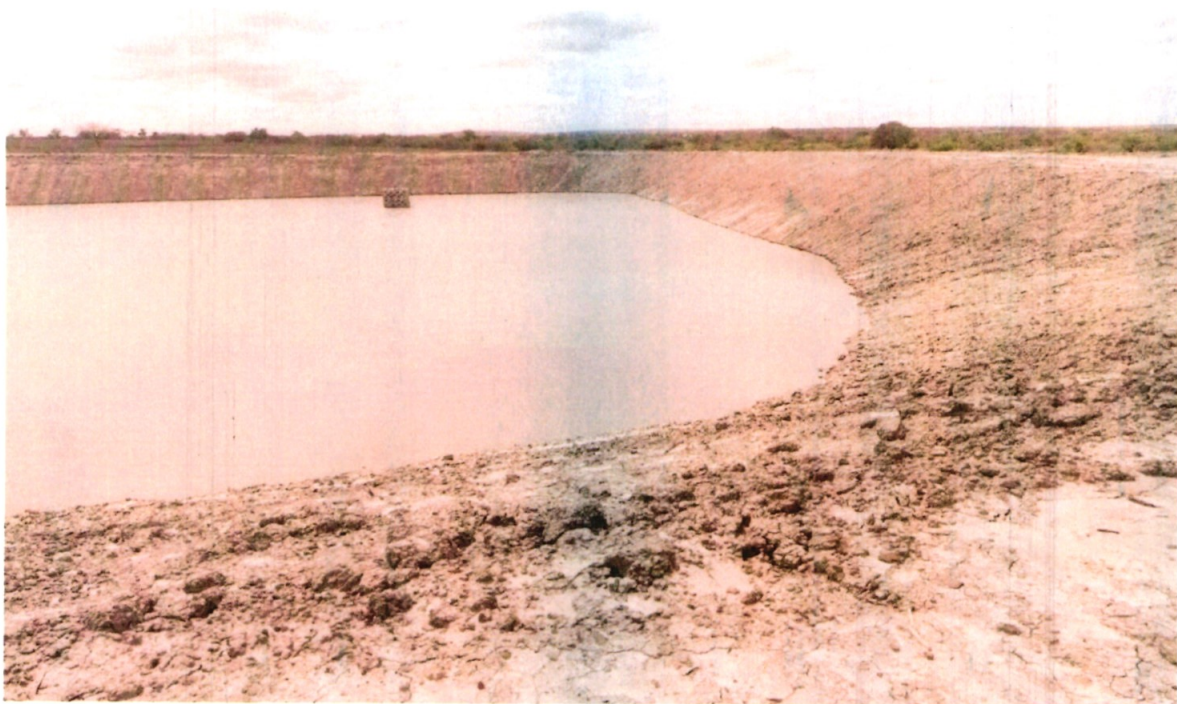
Expansion and distillation of Kakindu dam in Ndavaya ward
