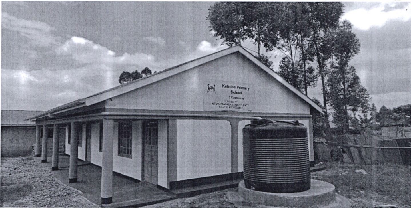
Riyabe Primary School - Construction of Construction of 2Nr. Classrooms @ Kshs. 3,000,000
