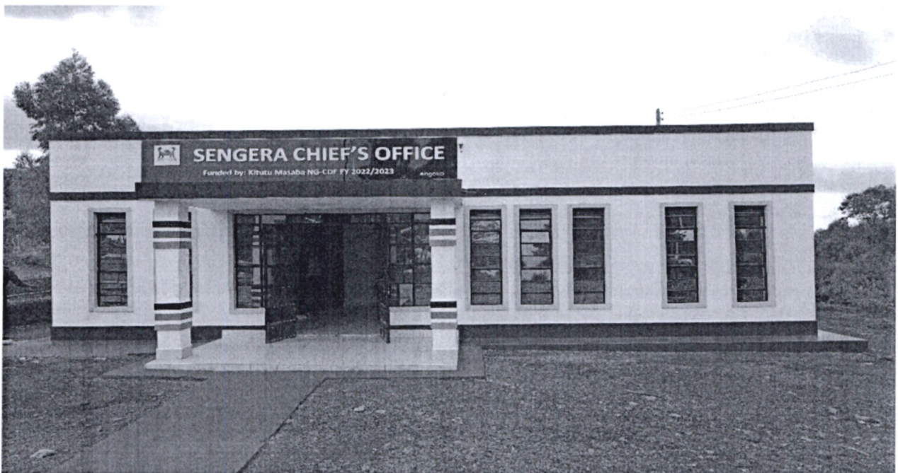
Sengera Location Chiefs Office: Construction of 5 roomed chiefs office @Kshs. 2,500,000
