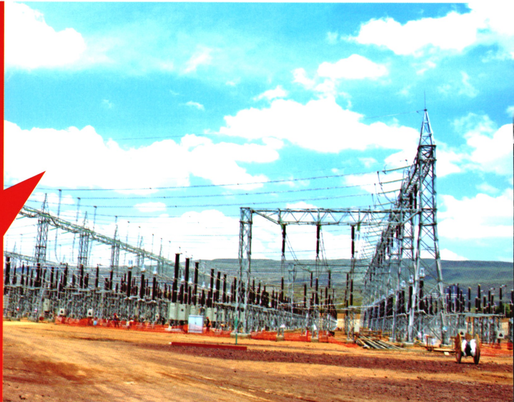
Ongoing works at Suswa - substation
