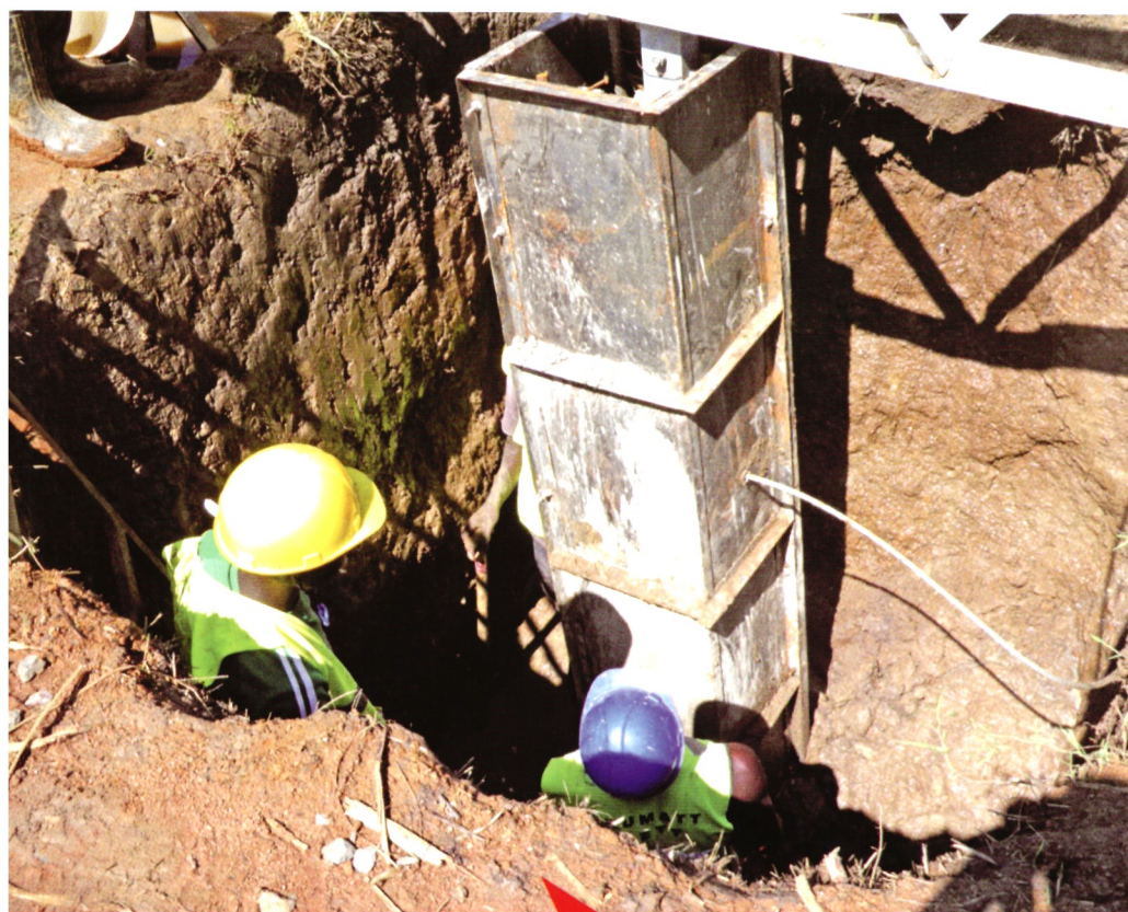
Ongoing foundation works along the Kisii Awendo project
