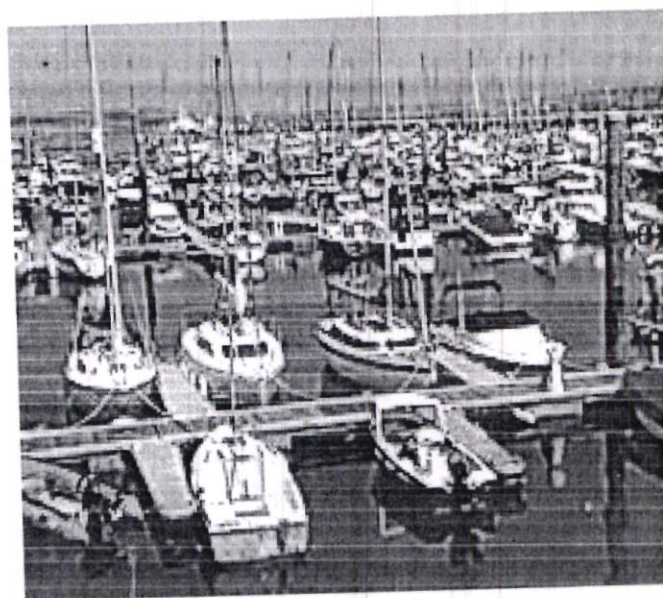
Figure 3: A small Marina at Brixham, Devon, England. The Vertical pilings attach the floating dock sections to the ground beneath the Water.
