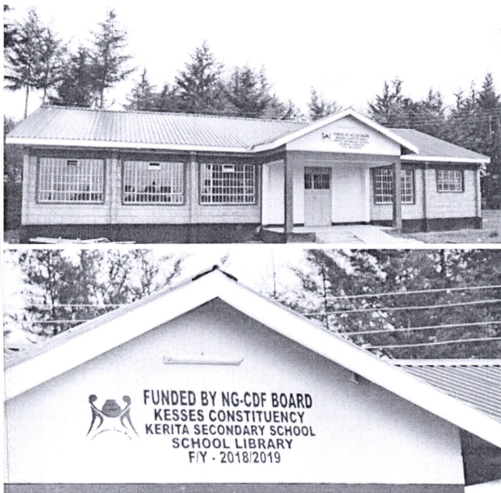
Construction of school library at Kerita Day Secondary School
