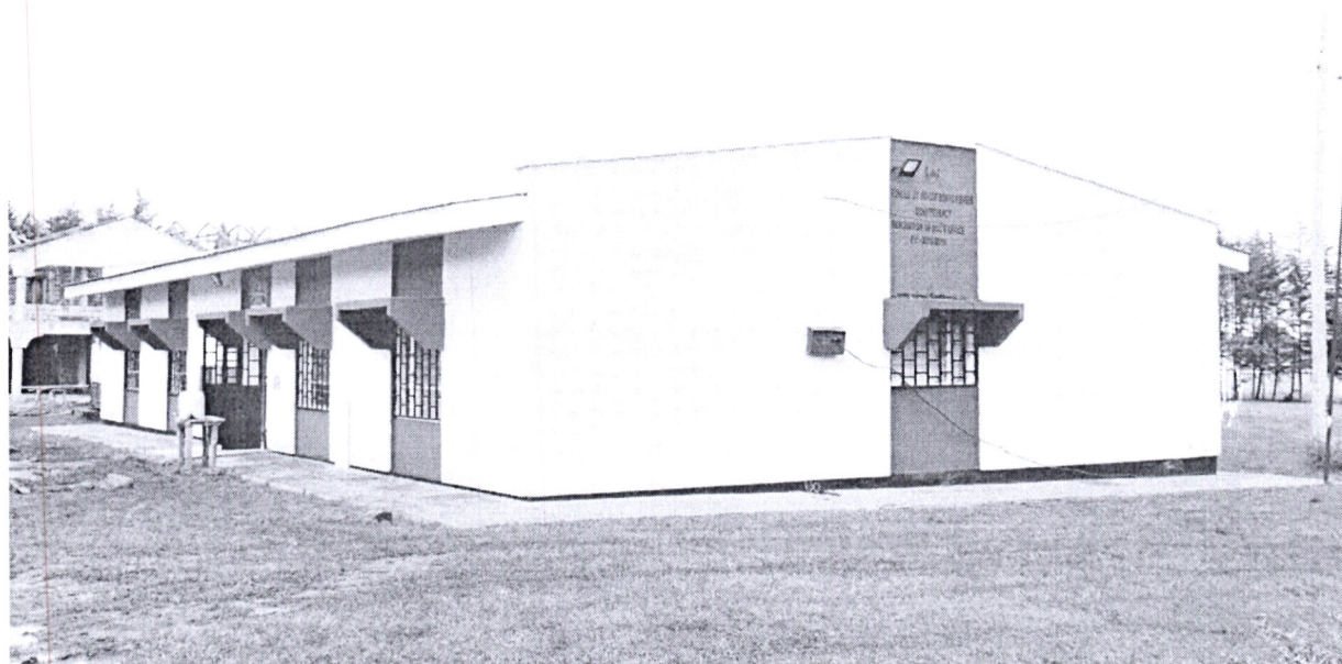
Renovation of DCC's office
