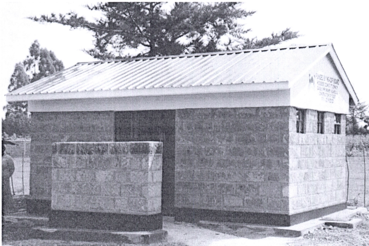
Construction of modern flush toilet for pupils with septic tank
