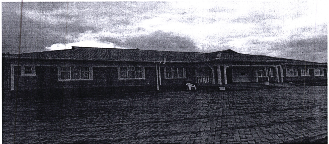
NG-CDF Office: Construction of the offices, furnishing and Fencing.
