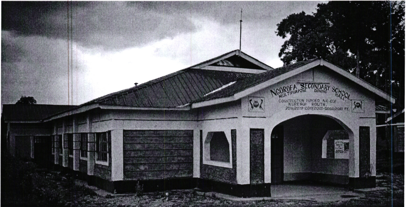
Ngorofa Secondary School | Construction of a multi-purpose hall
