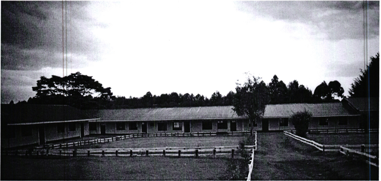
Olunguruone DEB Boarding Primary school Renovation of 8 classrooms
