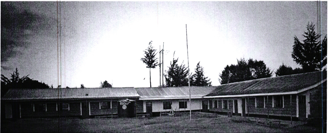
Sugutek primary school Renovation of 6 classrooms
