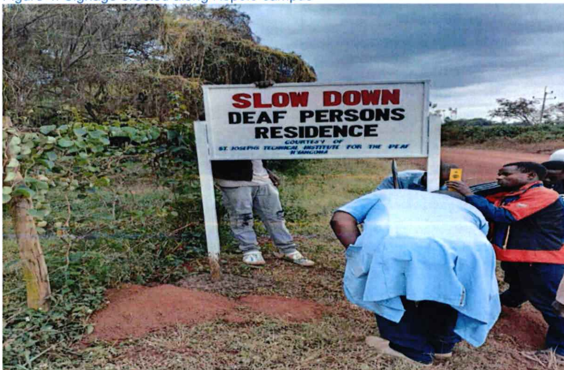
Figure 5: Trainees and trainers working on the signage along Nango- Nyang'oma road
