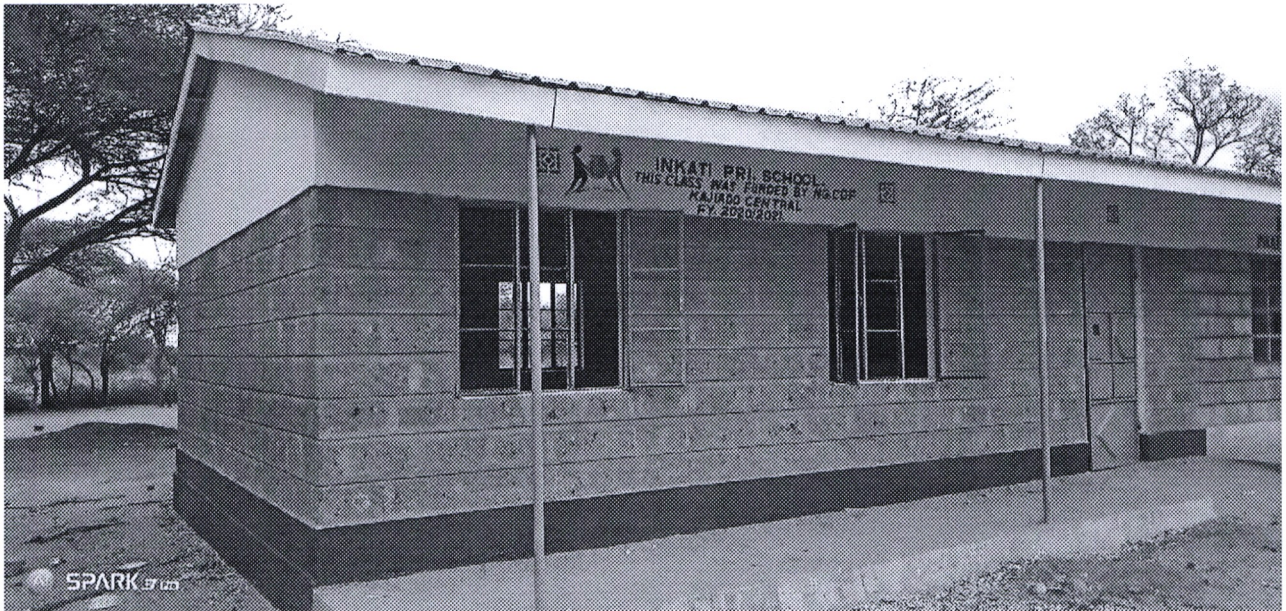
Fig 1. Classroom Construction at Inkati Primary School
