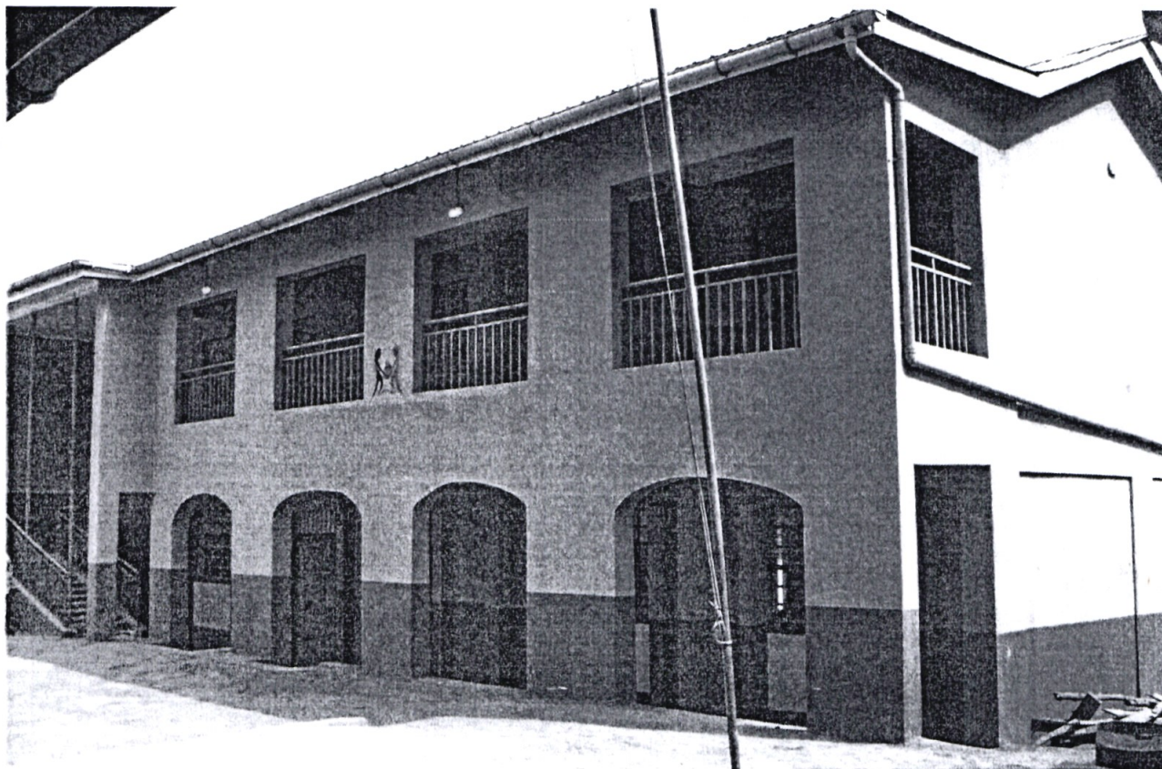
Construction of extension of classroom block at St. MarysKaimba Primary School
