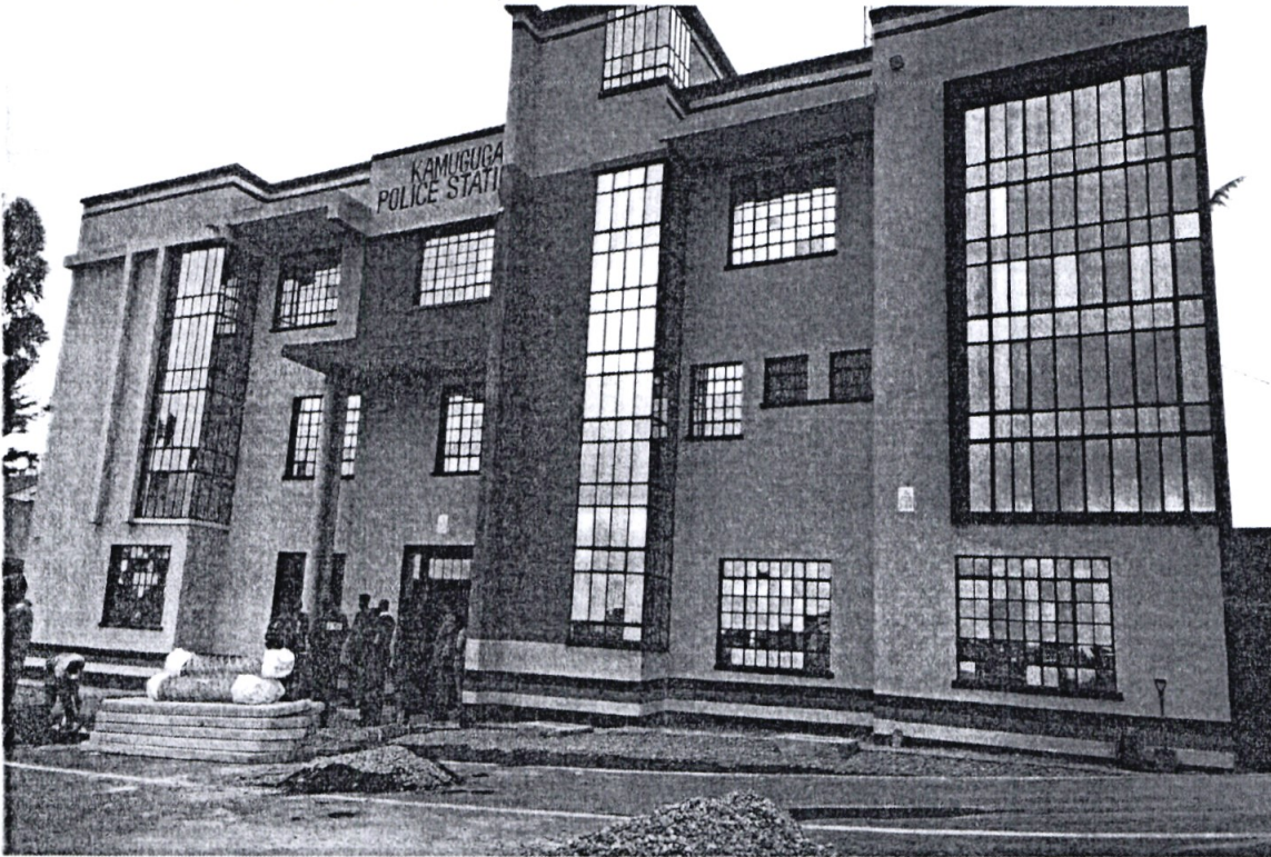
Above: The complete Kamuguga Police Station
