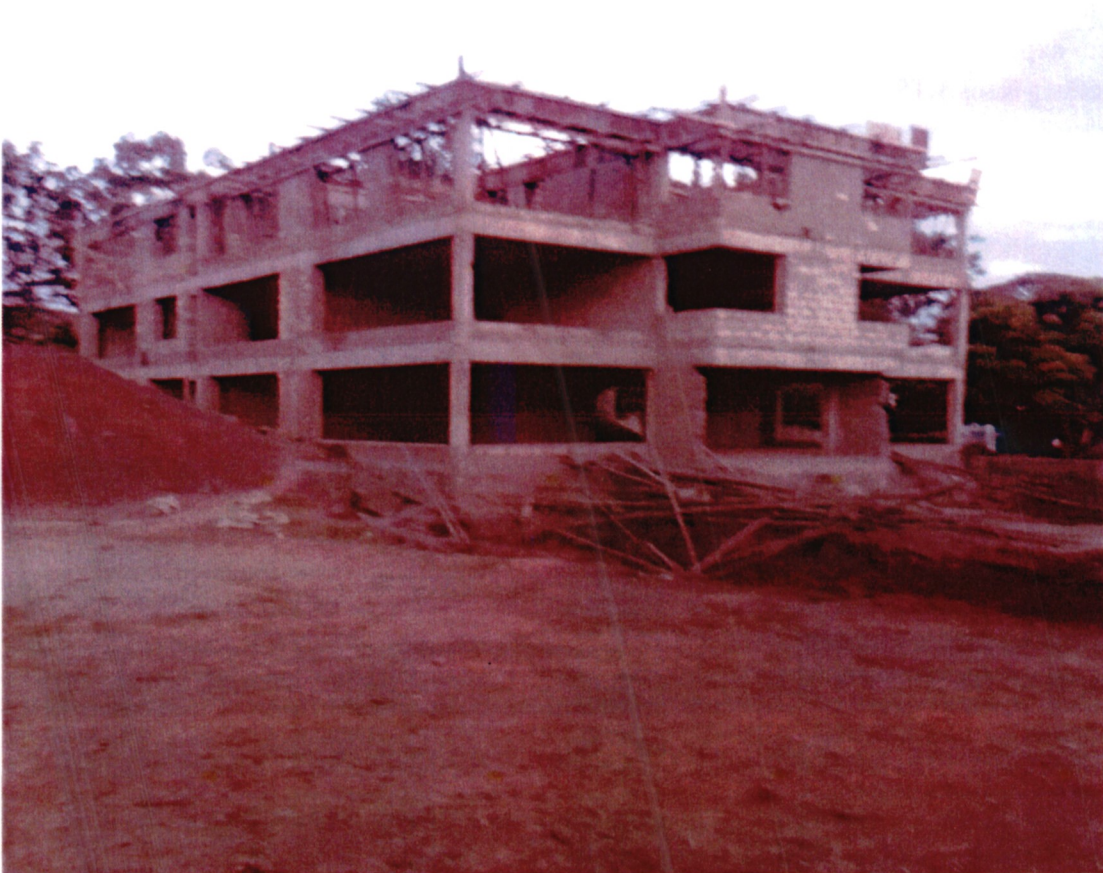
Fig. 1 on-going construction of Machakos TSC county office
