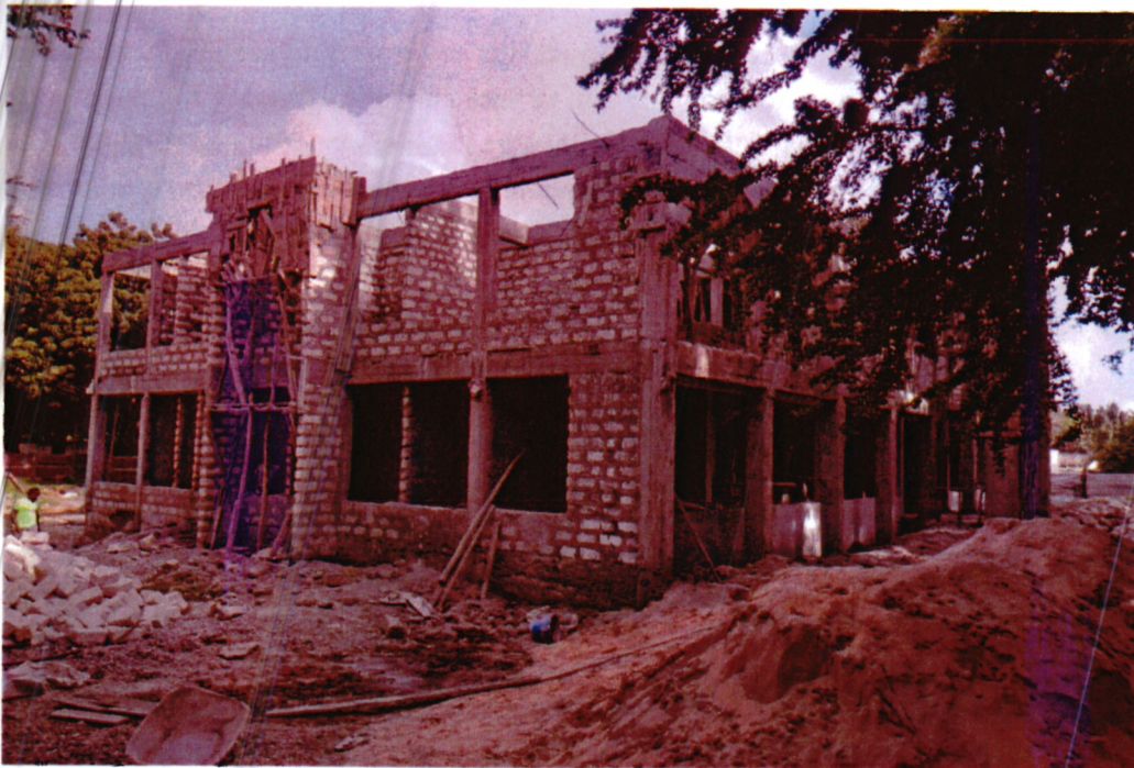
Fig.2 on-going construction of Kilifi TSC county office
