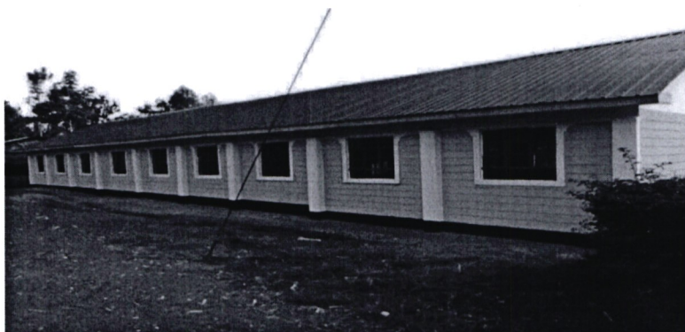
Fig 2. Construction of 3 classrooms at Chisaro Primary school
