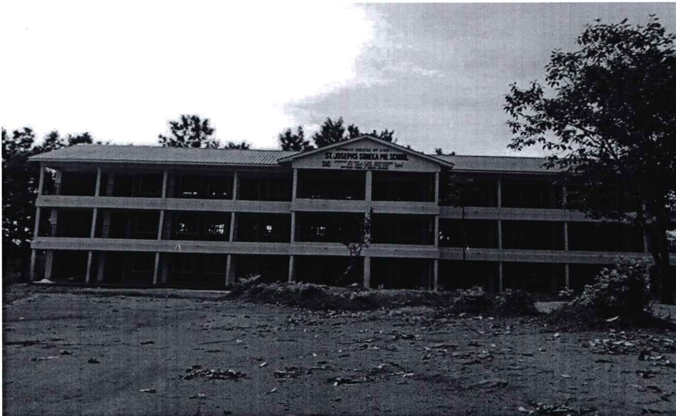
Fig 1. Construction of Suneka primary school
