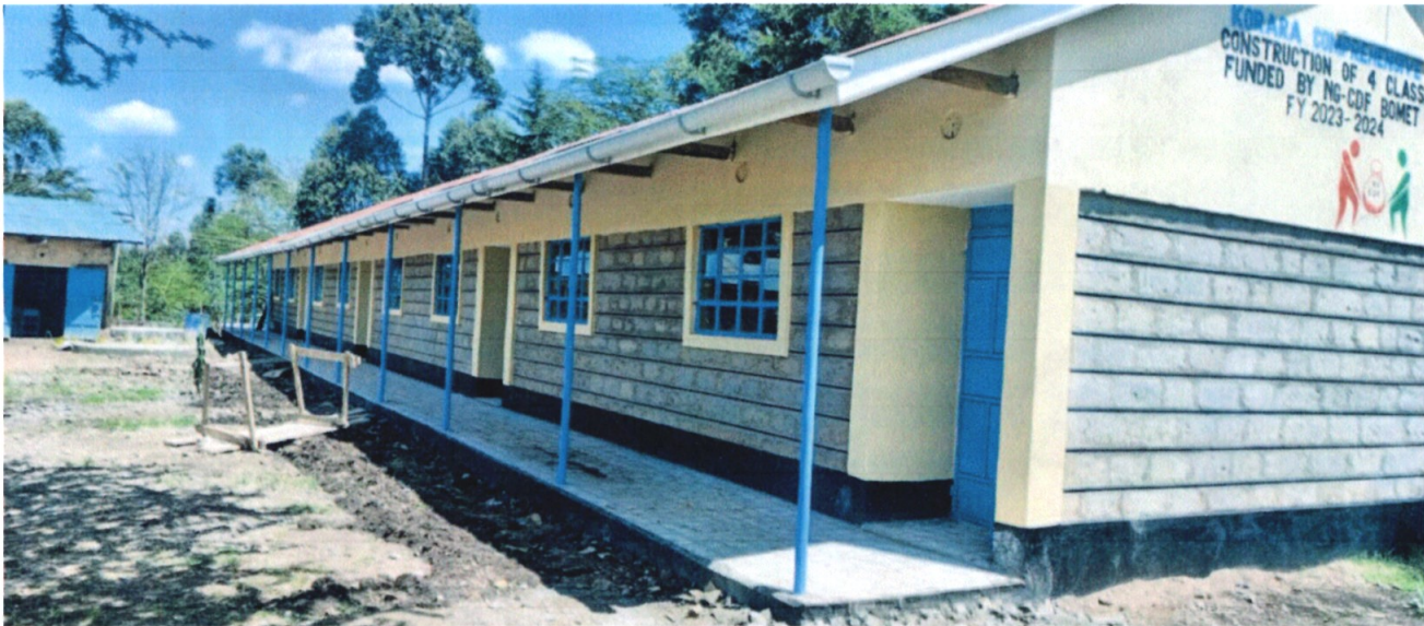
Fig 1.5 Photo of Complete 4 Classrooms at Korara Primary School
