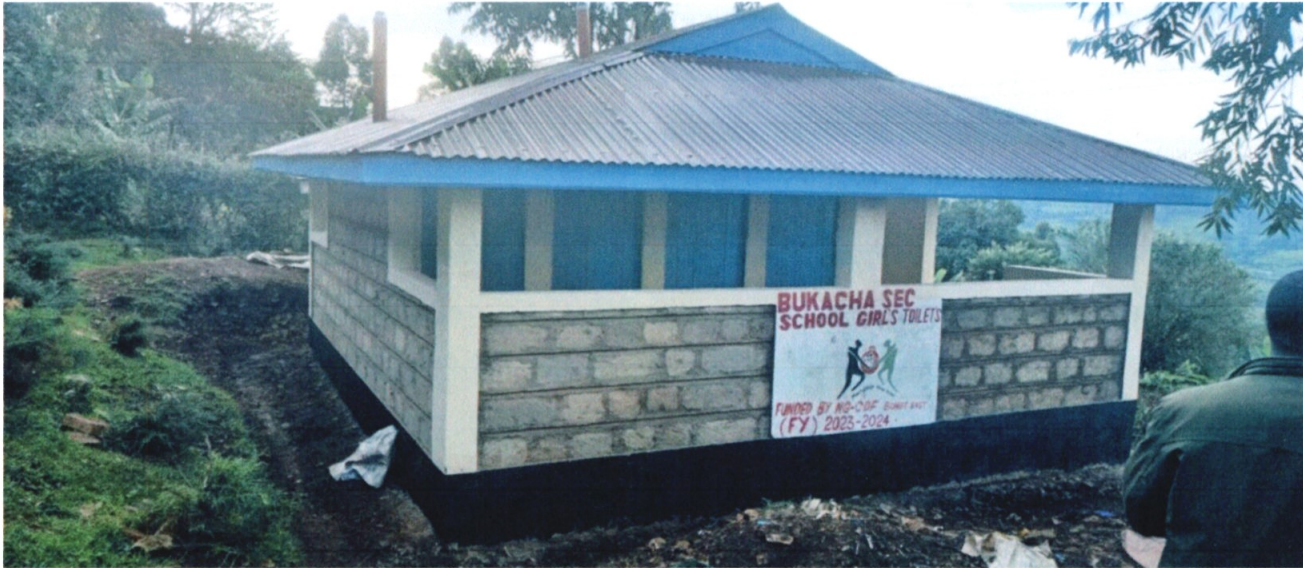
Fig 1.6: Photo of a Complete 8 Door Toilet at Bukacha Secondary School
