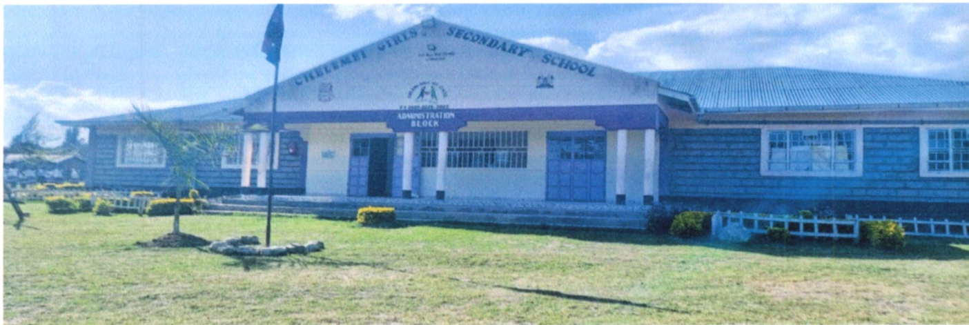
Chelemei girls secondary school administration block
