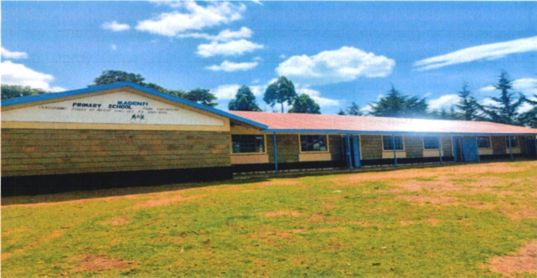
Fig 1.2: Construction to completion of 4 modern classrooms at Magenji Primary and Junior School.
