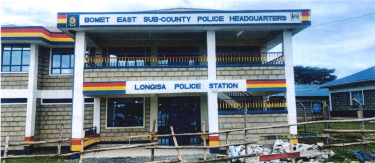
Photo of complete Bomet East Police Headquarters
