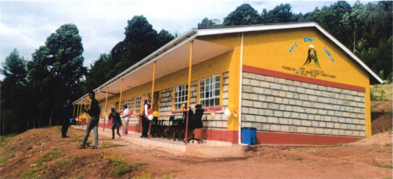
Fig 1.1 Construction to completion of 4 classrooms at kmtc bomet
