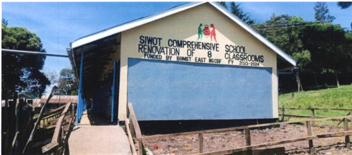
Fig 1.4 Photo of complete Renovation of 8 classrooms at Siwot Primary School
