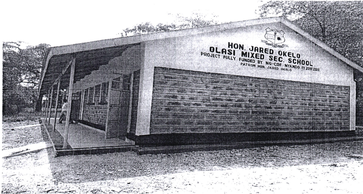
Two classroom tuition block at Olasi Mixed Secondary School
