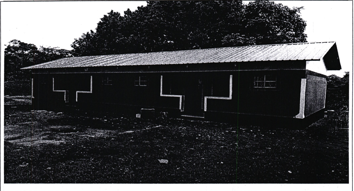
Fig. 2: Kipkomo Sub-County, 2 units AP houses
