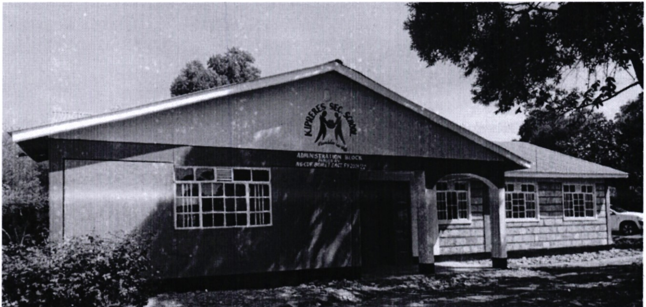
Bomet East NGCDF Office, F/Y 2022-2023, Construction of Administration Block
