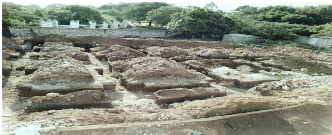
Figure 50: Foundation of the new accommodation rooms
