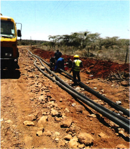
Excavation for laying of the 17 km pipel 1
