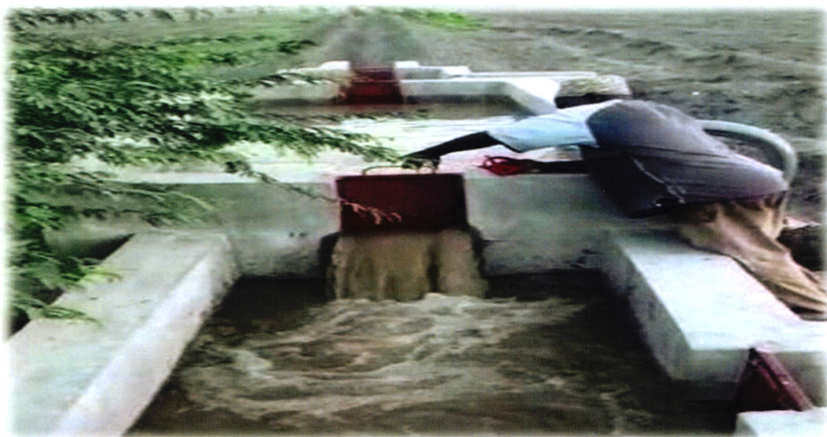
Figure 51: Water canal and distribution box at Boji
