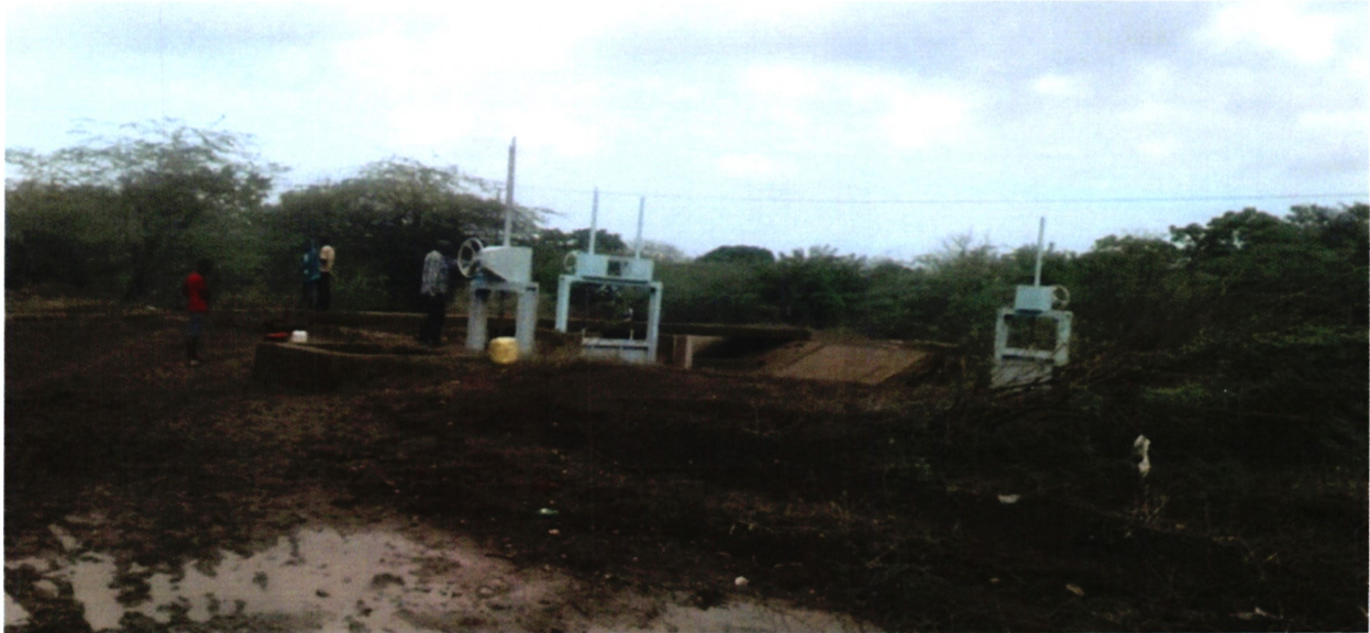
Repair of canal regulator gates at Hewani
