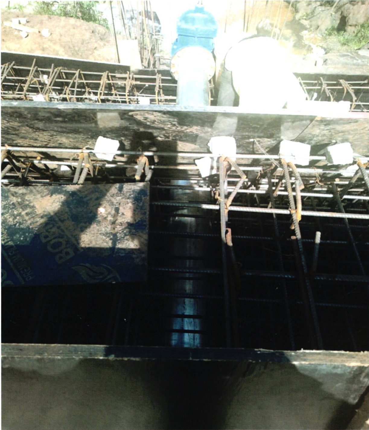
Figure 47: Gaitega Small Holder project water intake piping and reinforcement fixing works ongoing
