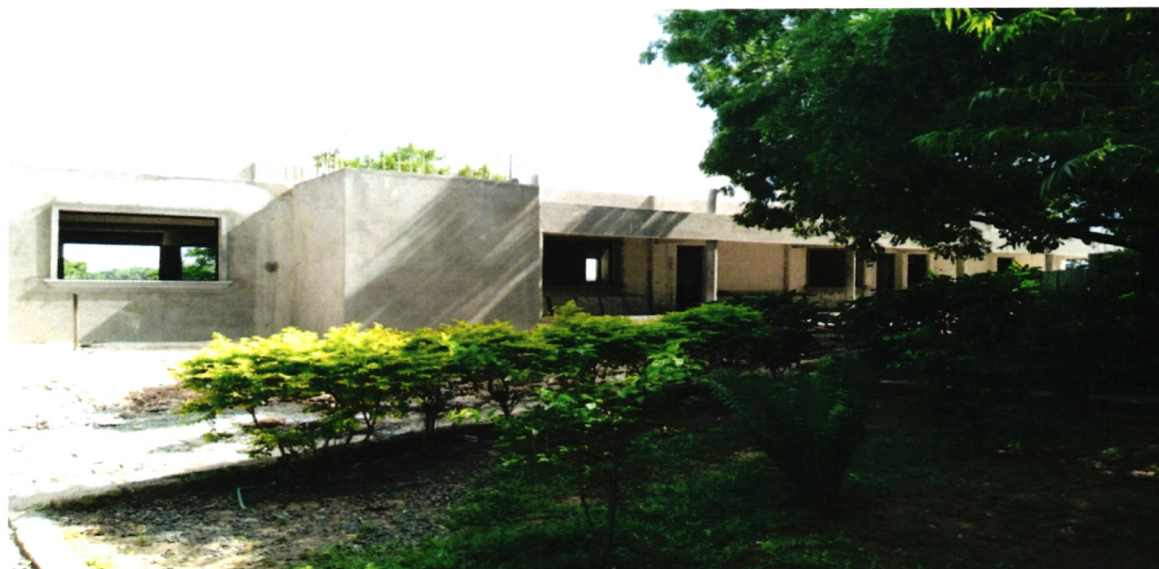
New conference facility under construction
