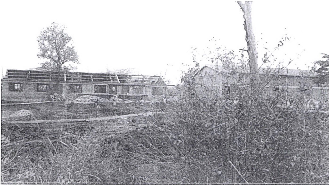
Front View of Instant Porridge and Yoghurt factory buildings
