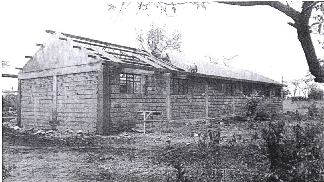
Back View of Yoghurt Factory Building
