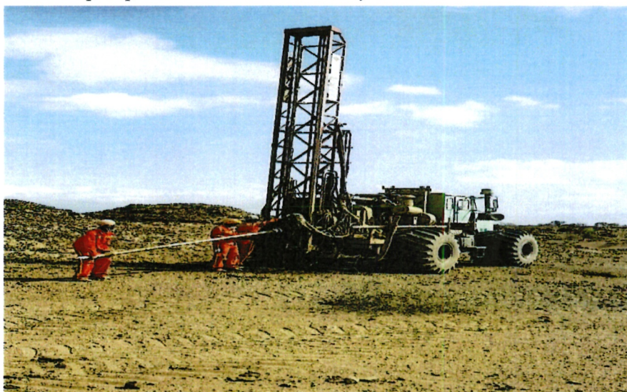
Drilling of shot hole during 2D seismic data acquisition in Block 14T
