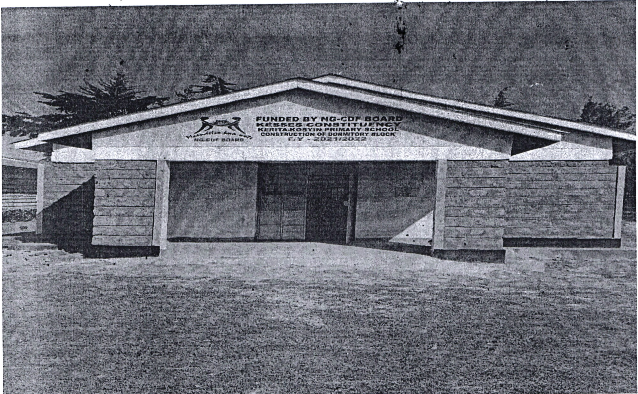
Kerita kosyin primary school – construction of dormitory
