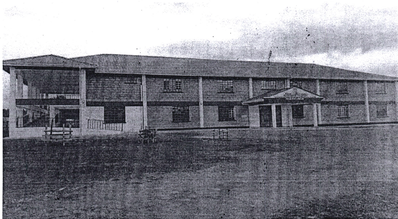
Racecourse secondary school – construction of administration block
