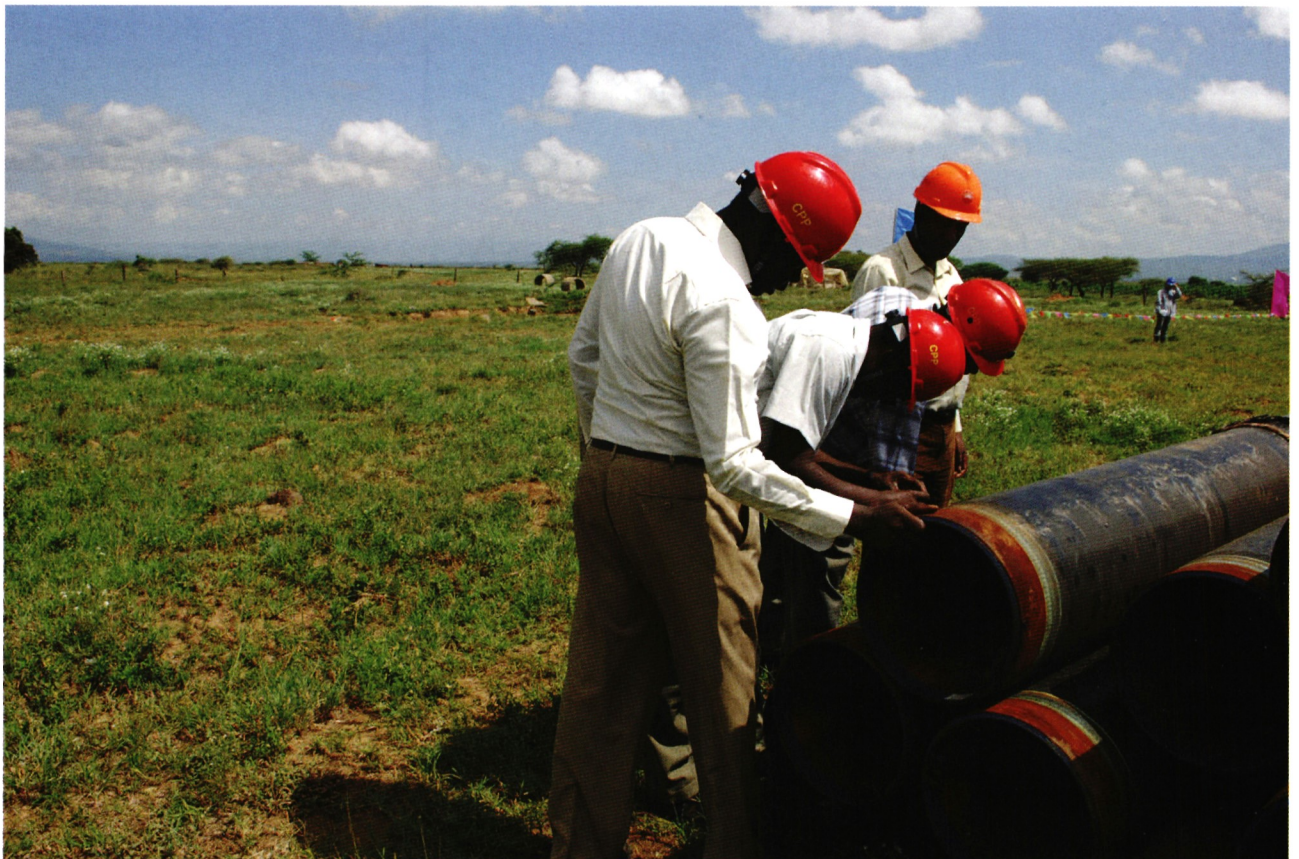
KPC engineer checking on integrity of pipeline
