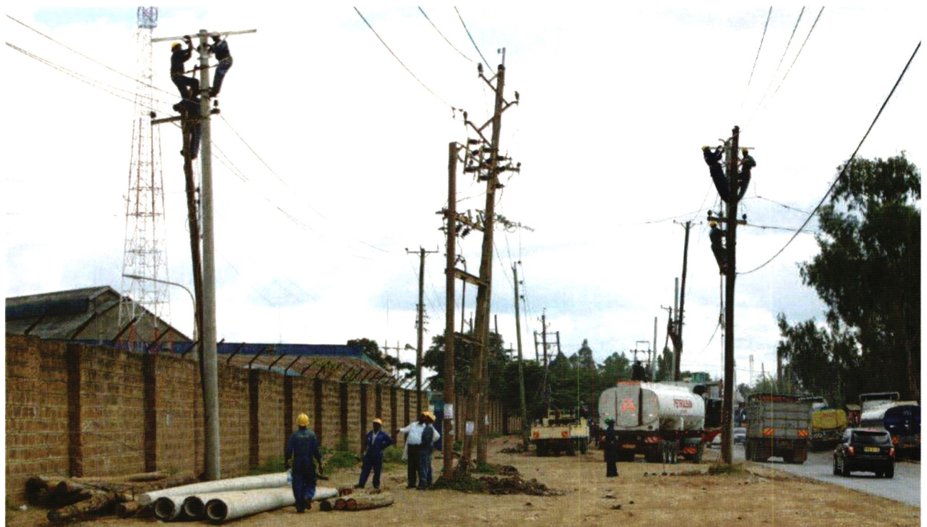
Kenya Power technicians carry out extensive work on the power infrastructure in Nairobi West as part of Operation Boresha Stima Viwandani in May 2014.
