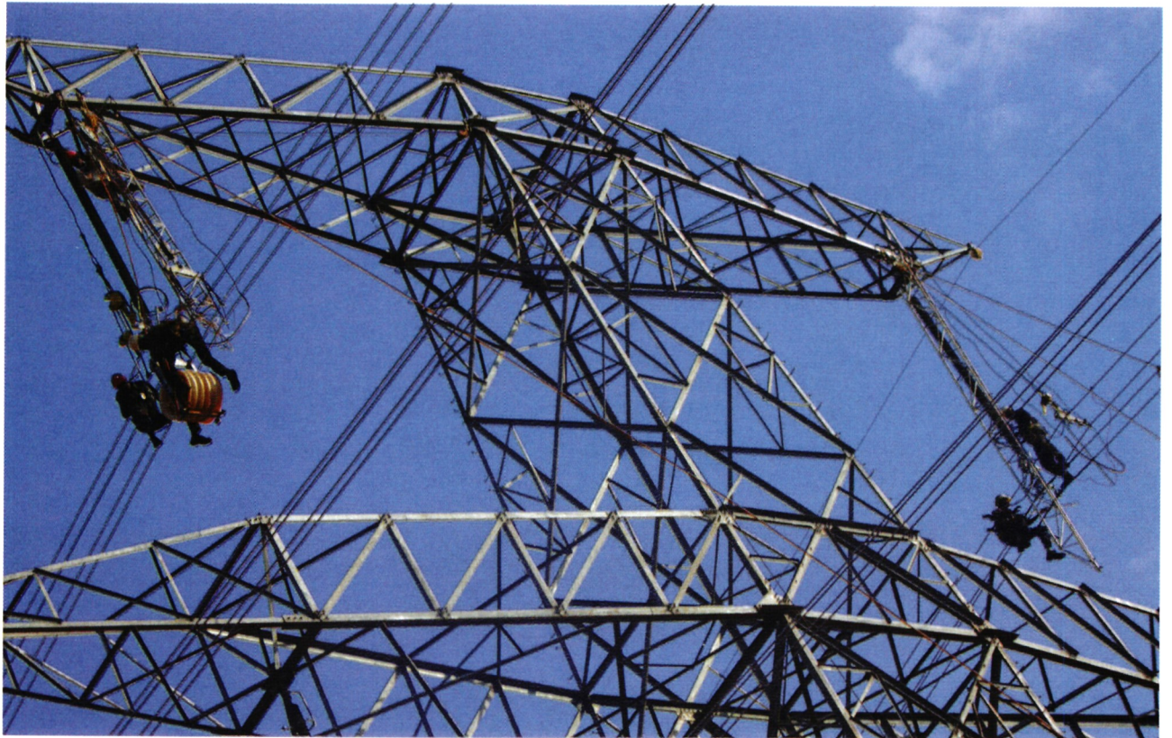
Ongoing stringing works along the 400kV Mombasa- Nairobi Transmission Project.
