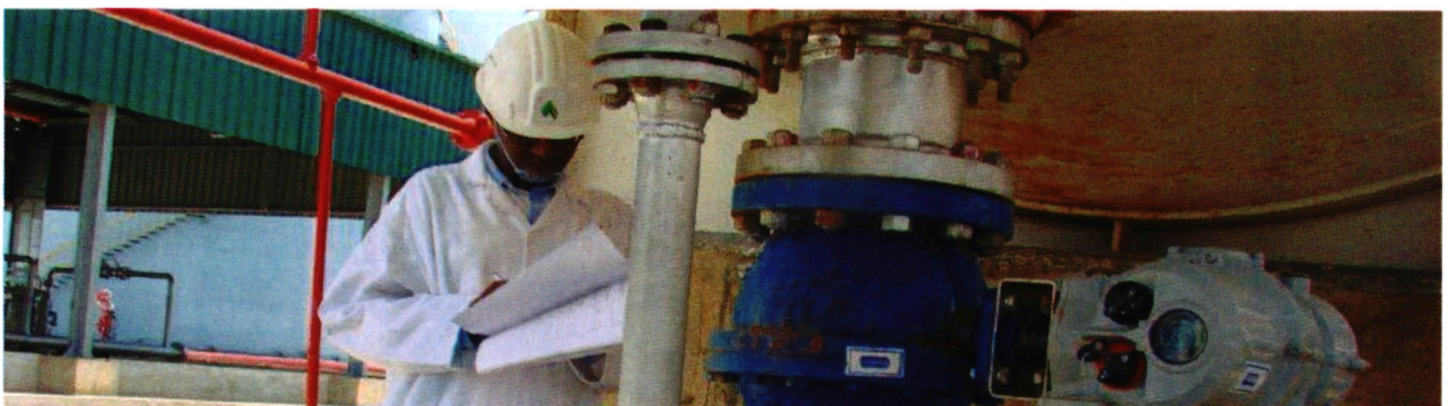
ERC officer inspecting a gas and oil installation
