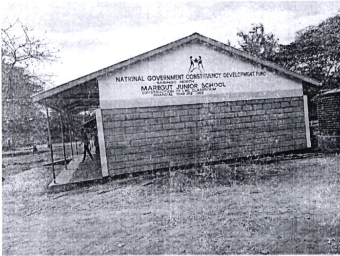
Complete construction of 1 classroom at Maregut Primary School
