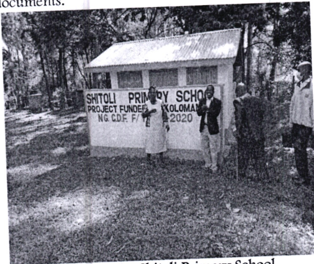
Emergency Project – Shitoli Primary School
