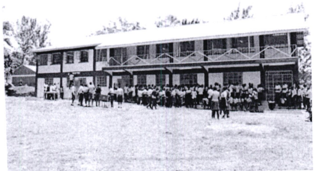
Shikokho Secondary School- Construction of a modern Administration
