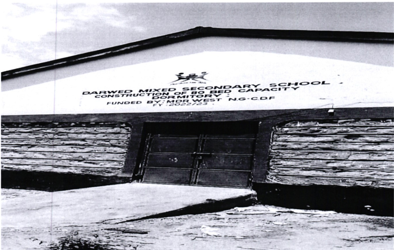
Construction of Dormitory at Darwed Mixed Secodary School. The dormitory has provided much needed accommodation and increased enrolment in the school.
