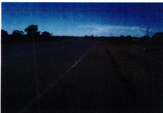
Picture 4: Completed road- Bondo-Misori road (August 2014)
