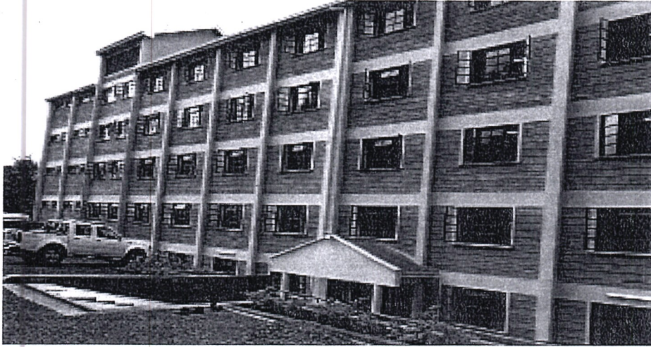
Hostel Block phase 1(Wing 1)
