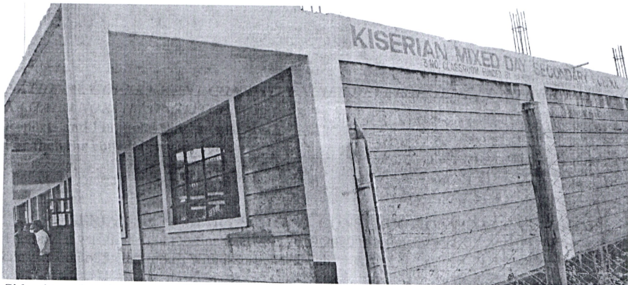
Side view of project
