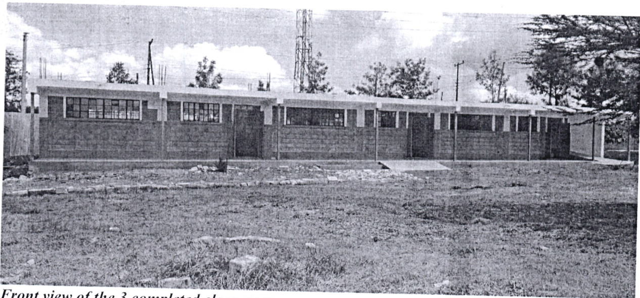
Front view of the 3 completed classrooms
