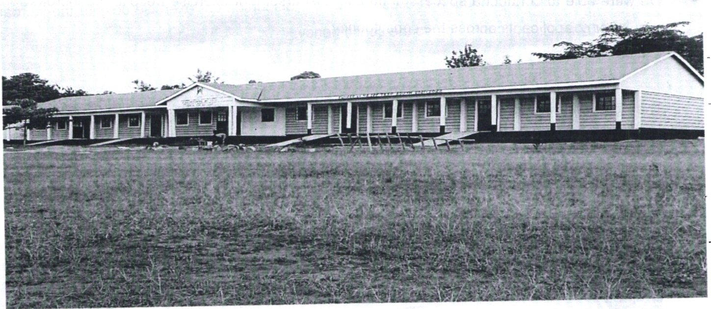
Figure 2: St. Pius Katelenyang Primary School – Construction of 4 no. classrooms with Administration Block
