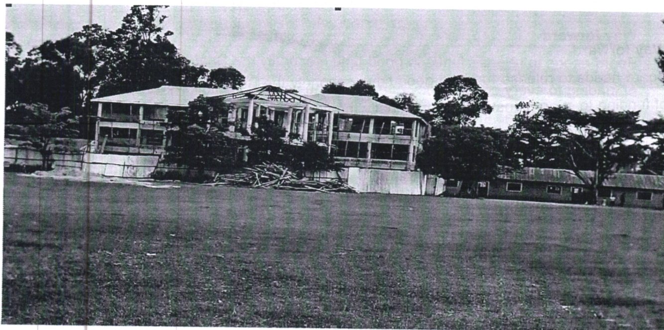
Figure 4 Ongoing two-storey building at Kaliwa Primary School
