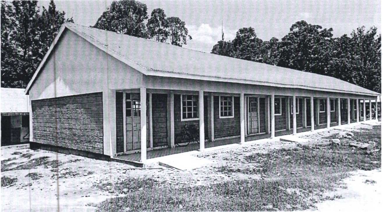
Figure 1: Kamunoit Primary School – Construction of 4 no. classrooms
