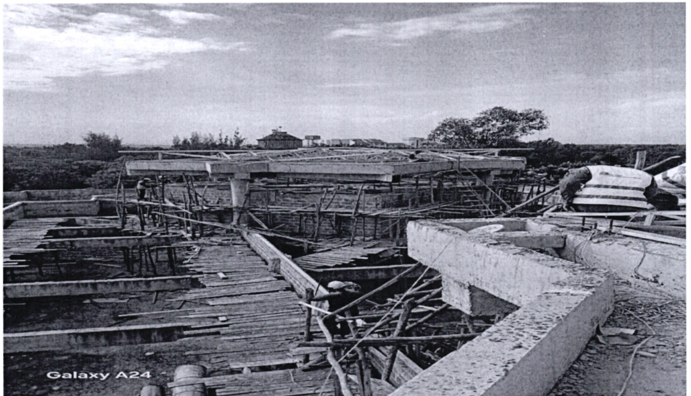
Installation of the roof for the Ultra-Modern Library
